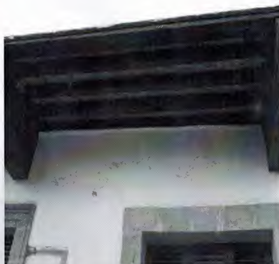
PLATE 36: The wooden construction of the base of the cumba at Sacakli Ev.
