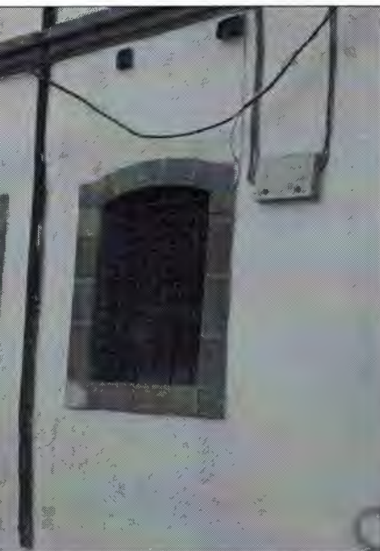
Two small doors transformed to windows on the front façade
