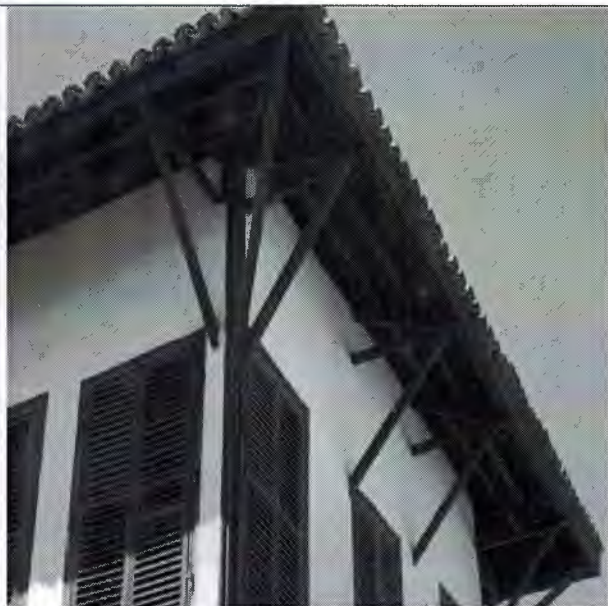
PLATE 38: The long Eaves of the Sacakli Ev made of wood.
