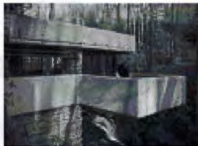
Fig 4.11 Frank Lloyd Wright's Kaufman house showing its cantilever ( www.architecture.about.com/buildingparts/cantilever )
