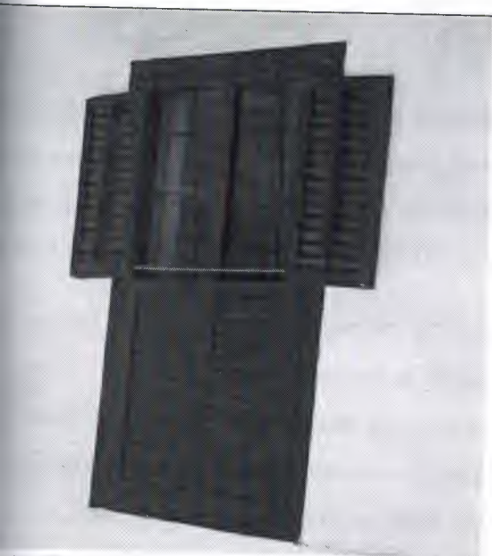
PLATE 53: The modified British window which has a single fold adopted from the Ottoman style which uses two folds
