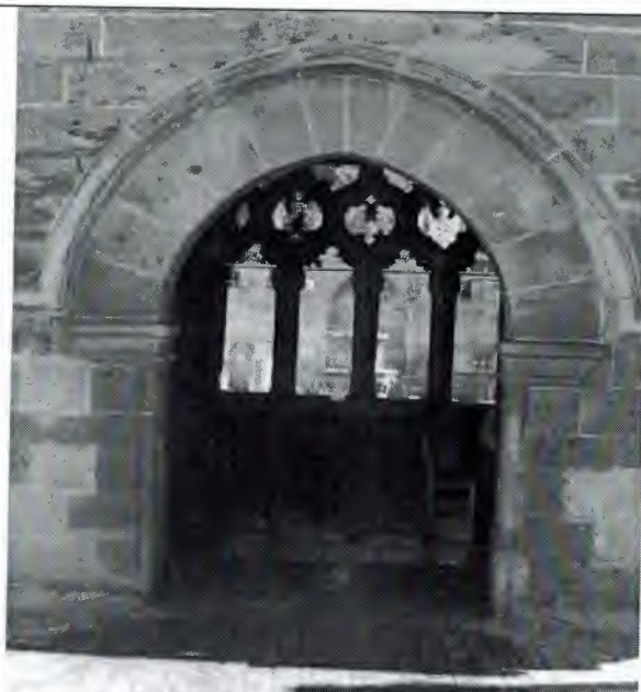
PLATE 18: The pointed gothic arched door with capping on both sides of the door frame and a stone decoration above
