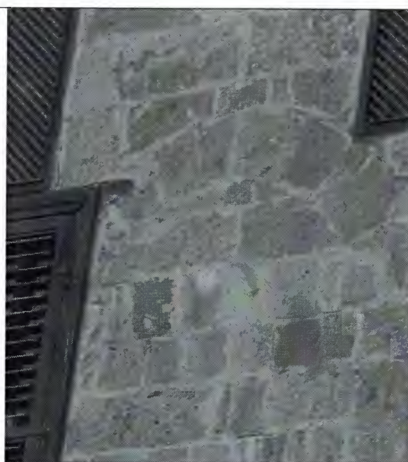
PLATE 6: Trace of an opening at a point in time which was blocked.
