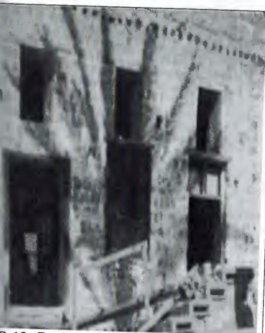
PLATE 13: During the same restoration work, small windows for lighting were added on the first floor.
