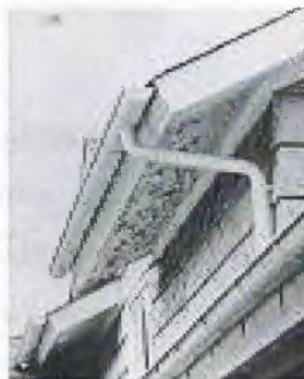
Fig 4.12 The eave of a building ( www.architecture.about.com/od/buildingparts/eave )
