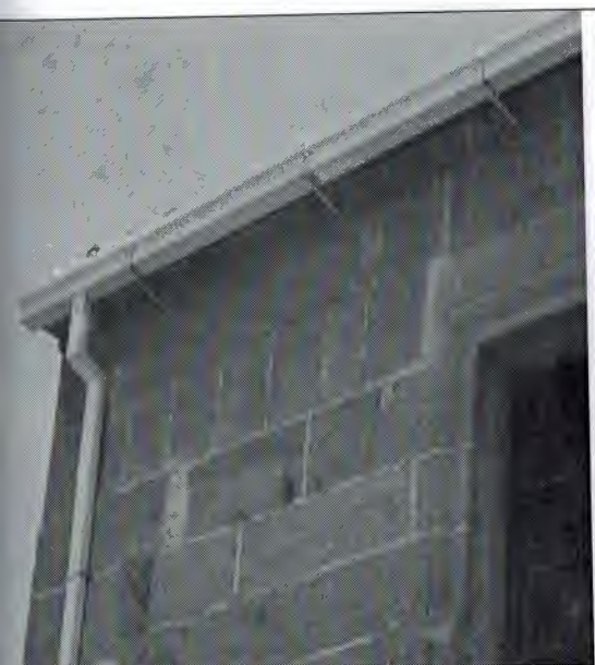
PLATE 23: The eave of the Lapidary Museum, with modern addition of aluminium cladding.
