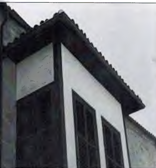
PLATE 7: The wooden eave of the Lusignan house, also seen are the wooden corner boards
