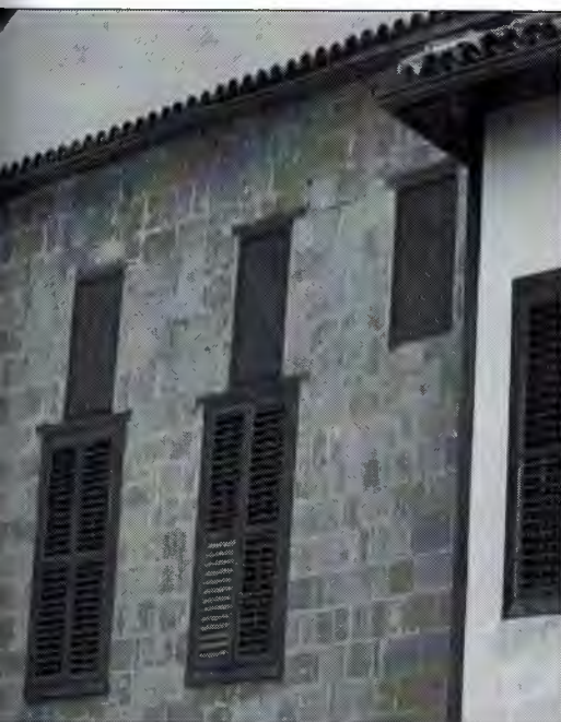
PLATE 5: Three small lighting windows on the first floor, which are added to resemble the original on the ground floor during restoration in 1996
