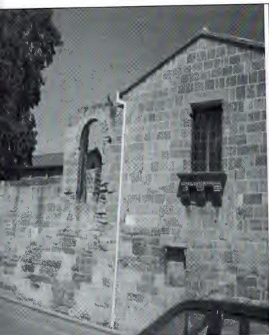
PLATE 21: The southern façade shows the arched window, the blocked window on the second floor and the semi circular archway.
