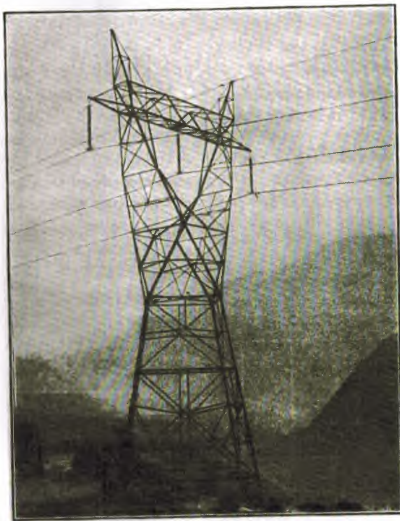
Figure 17 : Standard tower and sharp-thorned on single-circuit section of a dam with 287,000 volts transmission line.
