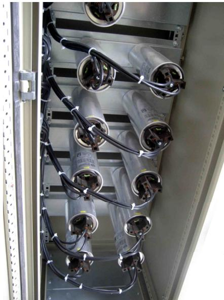
**Figure 3.4** Traditionally power factor capacitors in Bozkaya mine system
