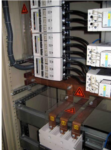
**Figure 3.5** Contactors and fuses
