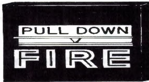
Figure 3.6. Manual pull box.
