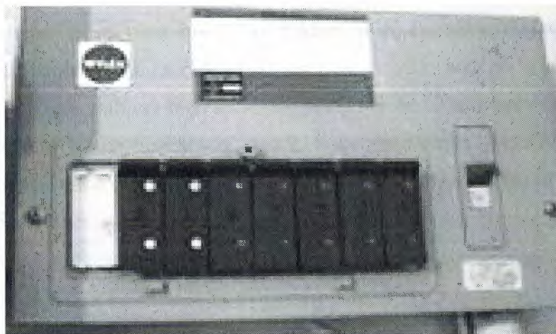
Figure 2.2: A Typical Fuse Box.
