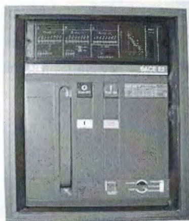
Figure 2.5: Front panel of a 1250 A air circuit breaker.
