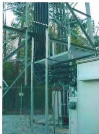
Figure 2.16 Using cables between radio antenna and tower
