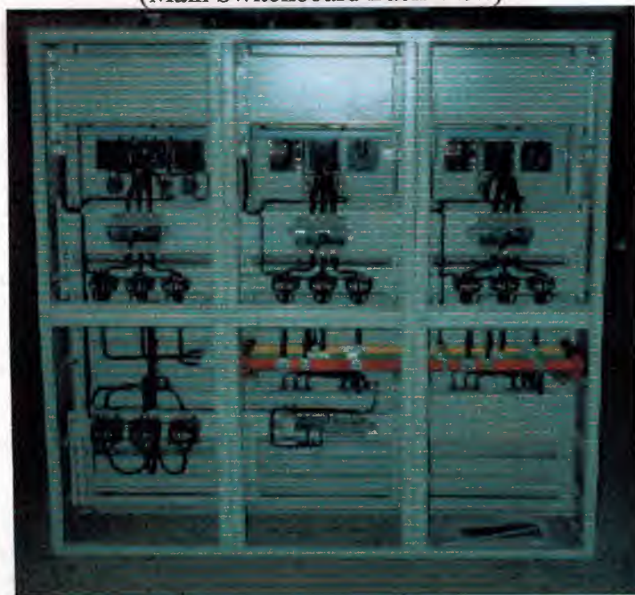
Figure-5- (Main Switchboard Back View)
