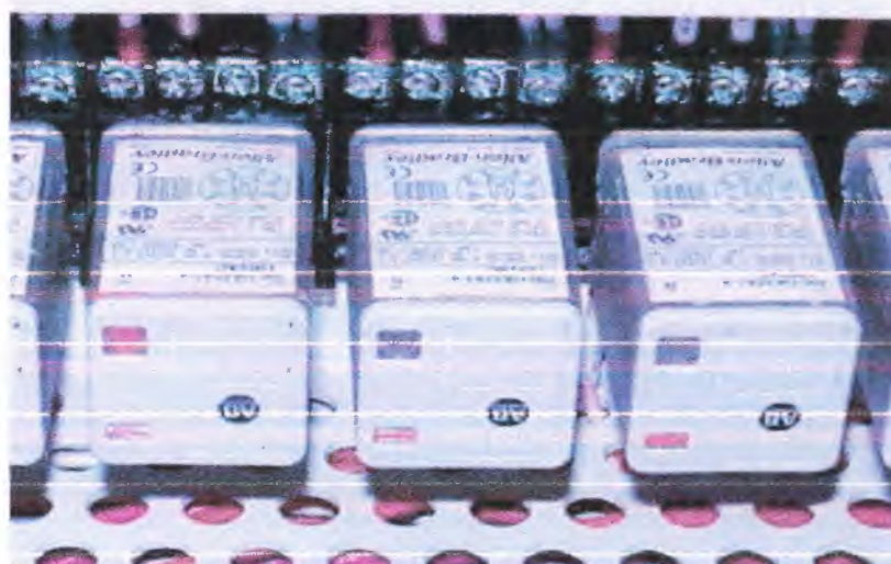
Figure 2.10 relays installed on a panel.
