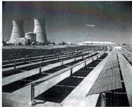
Figure 3.2 A 2-MW utility-scale photovoltaic power system co-located with a defunct nuclear power plant near Sacramento, California.
