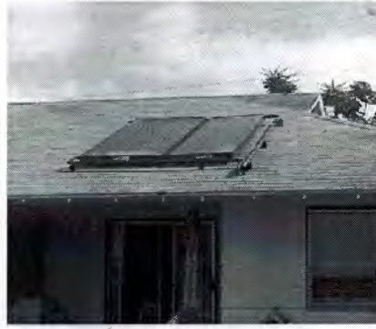
Figure 3.7 Flat-plate thermal solar collectors for providing hot water
