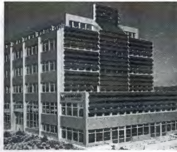
Figure 4.12 Scheidegger Building with photovoltaic facade near Bern in Switzerland
