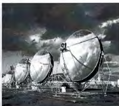
Figure 3.12 Two-axis tracking parabolic dishes collectors
