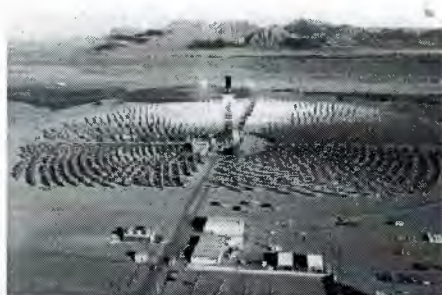
Figure 3.11 A central receiver system.
