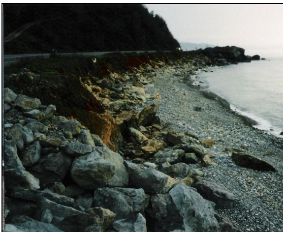
Figure 1. Waves are carving the bottom of the fillings.
