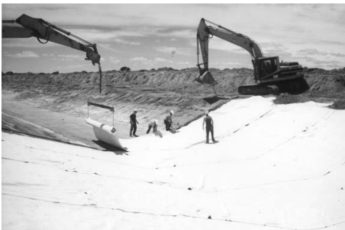
Figure 3. Installing the GCL.
