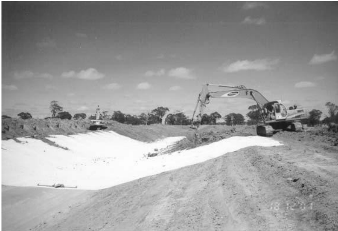
Figure 4. Burying the GCL.
