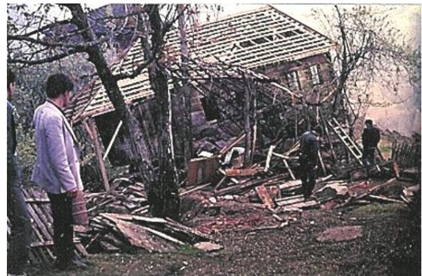
Figs. 6-7 Damaged and tilted houses with respect to vertical position due to landslide.
