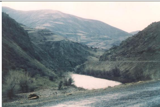
Figure 17 The abandoned Ispir Dam site Figure 18 Ispir reservoirs' landslides. due to landslides in its reservoir.
