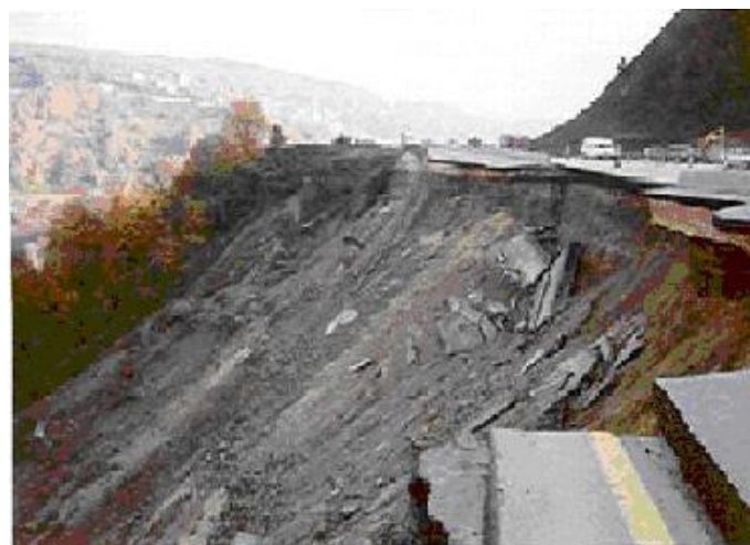
Figure 16 A landslide on Bolu-Istanbul highway which destroyed half of the highway.
