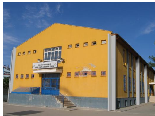
Figure 5. Existing primary school after strengthening with ESM
