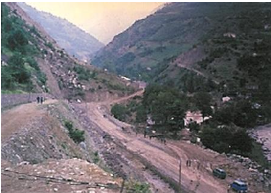
Figs. 12-13 Blocked road and a river which has changed its bed due to landslide
