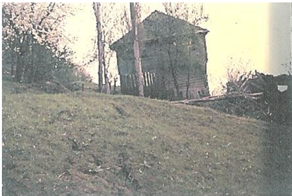
Figs. 6-7 Damaged and tilted houses with respect to vertical position due to landslide.
