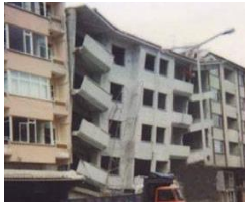
Figure 1. Totally collapsed RC building due to the architectural and design mistakes
