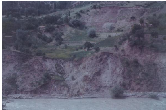
Figure 17 The abandoned Ispir Dam site Figure 18 Ispir reservoirs' landslides. due to landslides in its reservoir.
