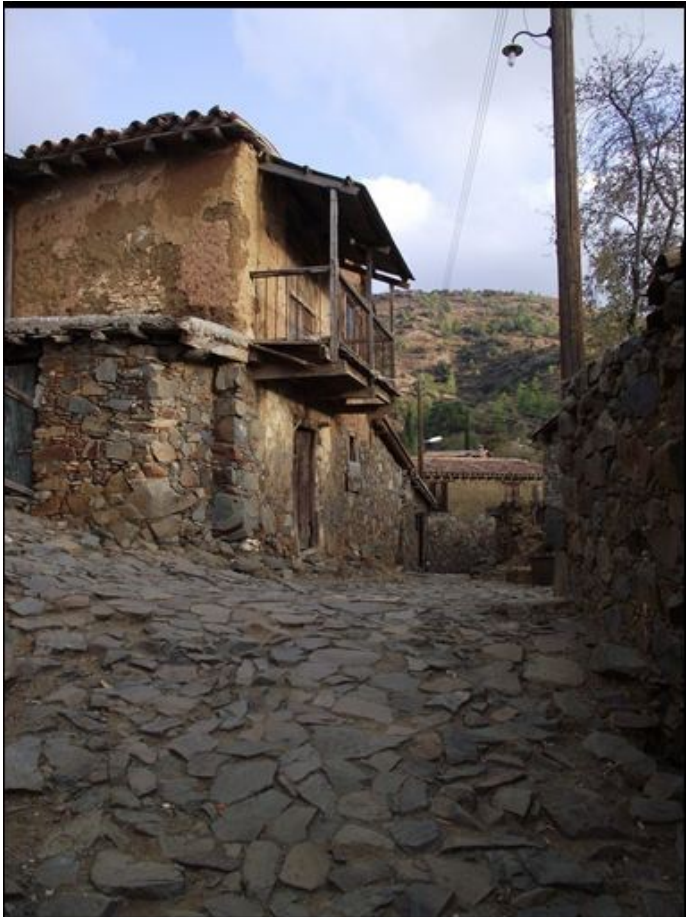
Figure 3.7 The Sample of Two Storey Rural House in Ottoman Period, Fikardü Village, Trodos. http://zsota.blogspot.com/2010/11/loni-valo-hal-biciklituraval.html
