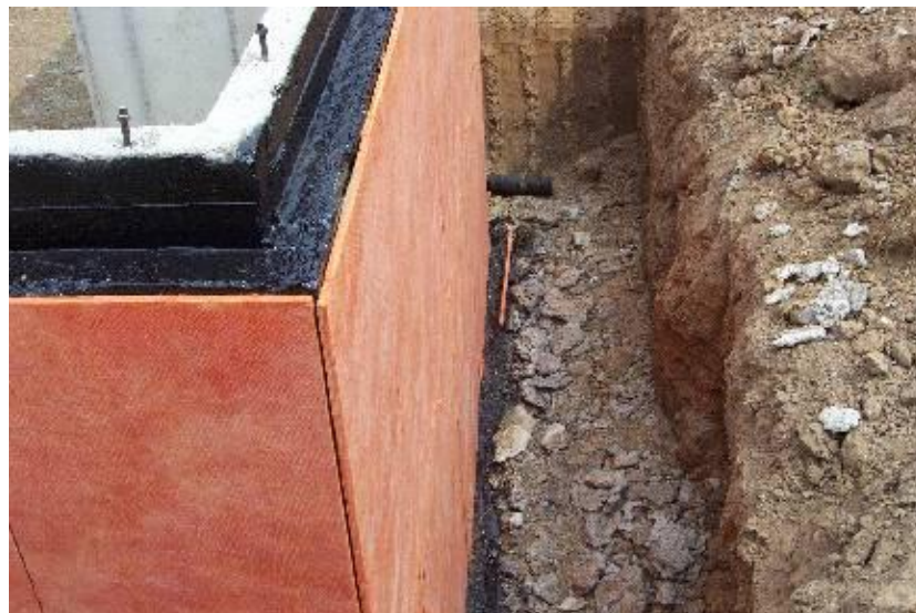
Figure 3.16: Insulating Basement Walls Externally [27].
