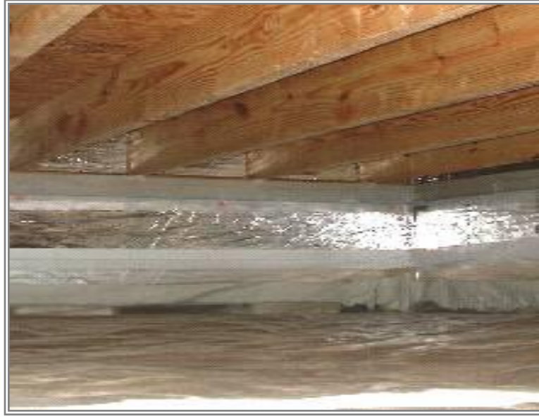
Figure 3.17: Adding Insulation on Basement Walls Internally [27].
