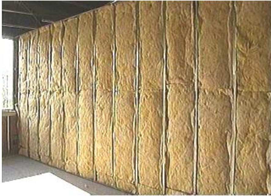
Figure 3.6: Wall Insulated Internally [27].
