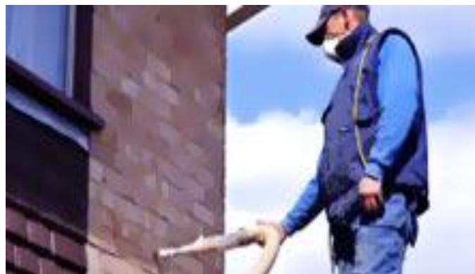
Figure 3.12: The Way to Insulate a Cavity Wall [31].
