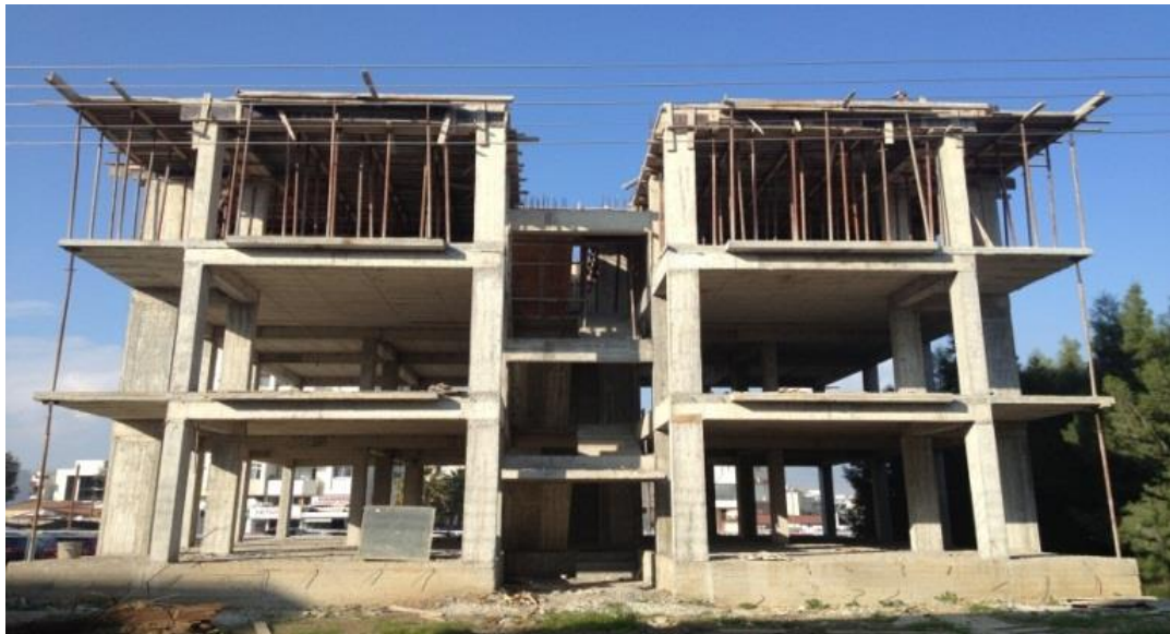
Figure 5.1 Rough Construction of Multi-Storey Reinforced Concrete Building Structure.
