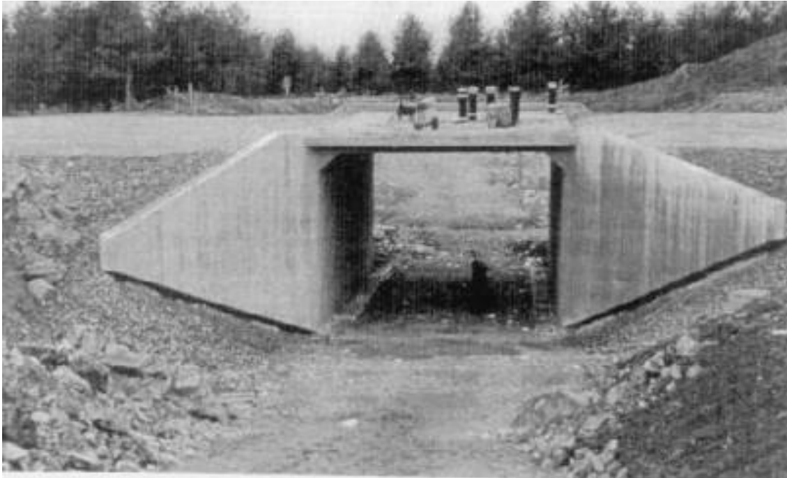
Fig 2.2: First Bridge with SCC in Sweden (Goodier, 2003)
