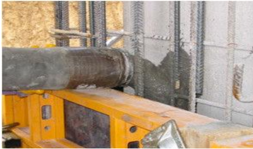
Fig 2.9: SCC Pouring process(Borimi, 2013)
