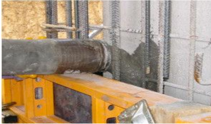
Fig 2.9: SCC Pouring process(Borimi, 2013)
