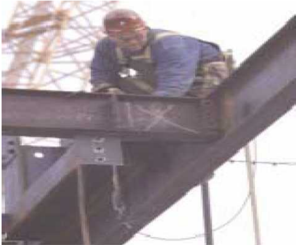
Figure 4.2: Typical Fall protection (Oregon OSHA, 2011)
