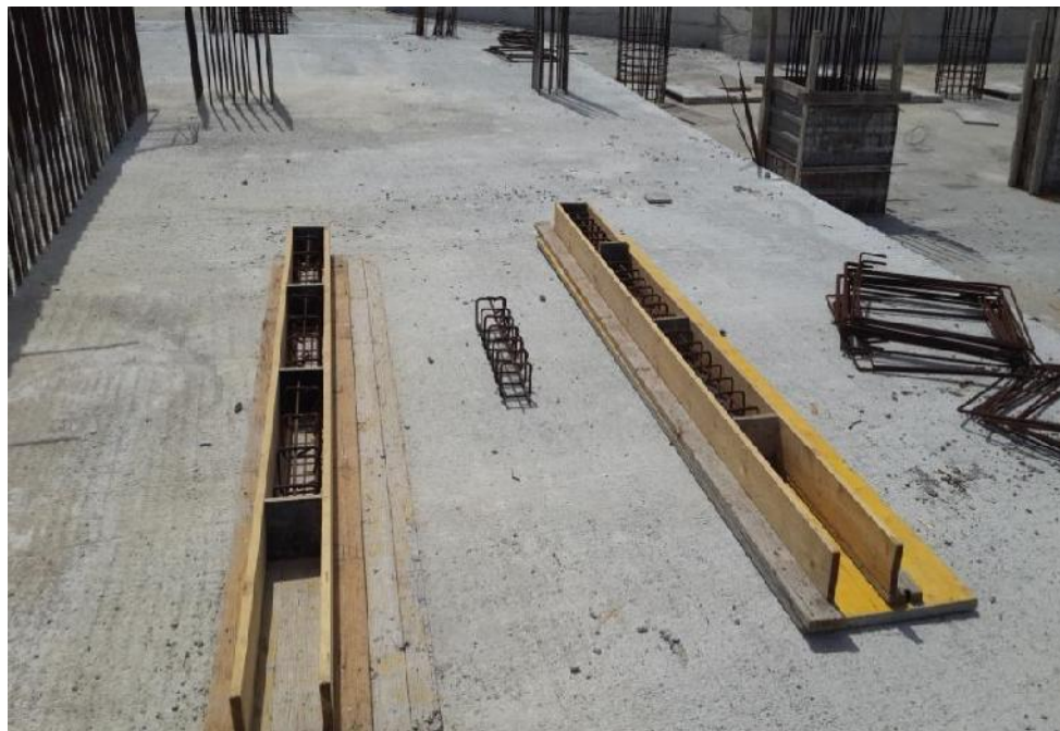
Figure 4.2: Moulds with Reinforcement before Casting
