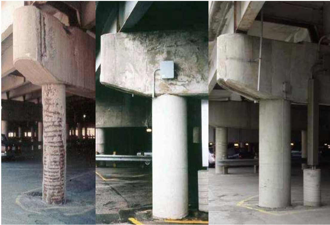
(a) Pre-repair (before repair) (b) After Repair (1996) (c) Seven Years after Repair (2003)
