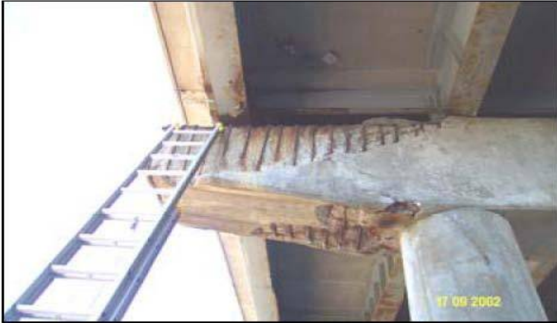
Figure 1.1: Typical Corrosion Damage Caused by Chloride-Contamination Leaks in Bridge Deck Joints [ http://www.structuremag.org/article.aspx?articleID=509 ]
