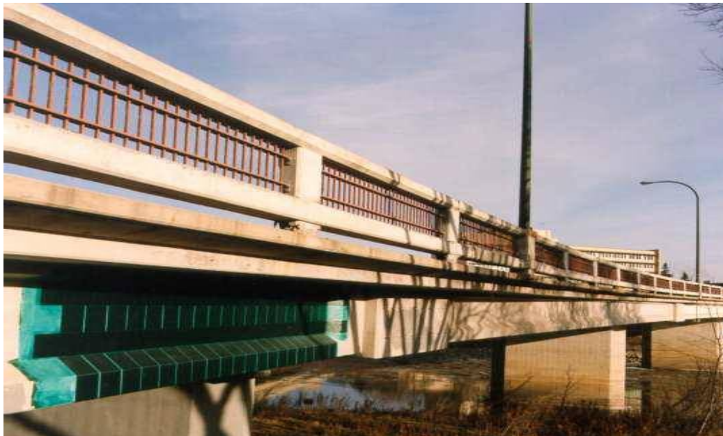
Figure 1.4: Shear Strengthening Inclined Orientation: Efficient Use of CFRP (Shahawy, 2010)
