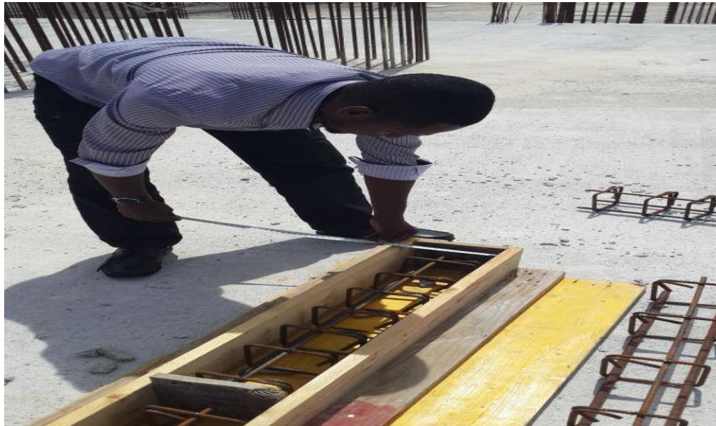
Figure 4.1: View of Group 2 Beam Reinforcement
