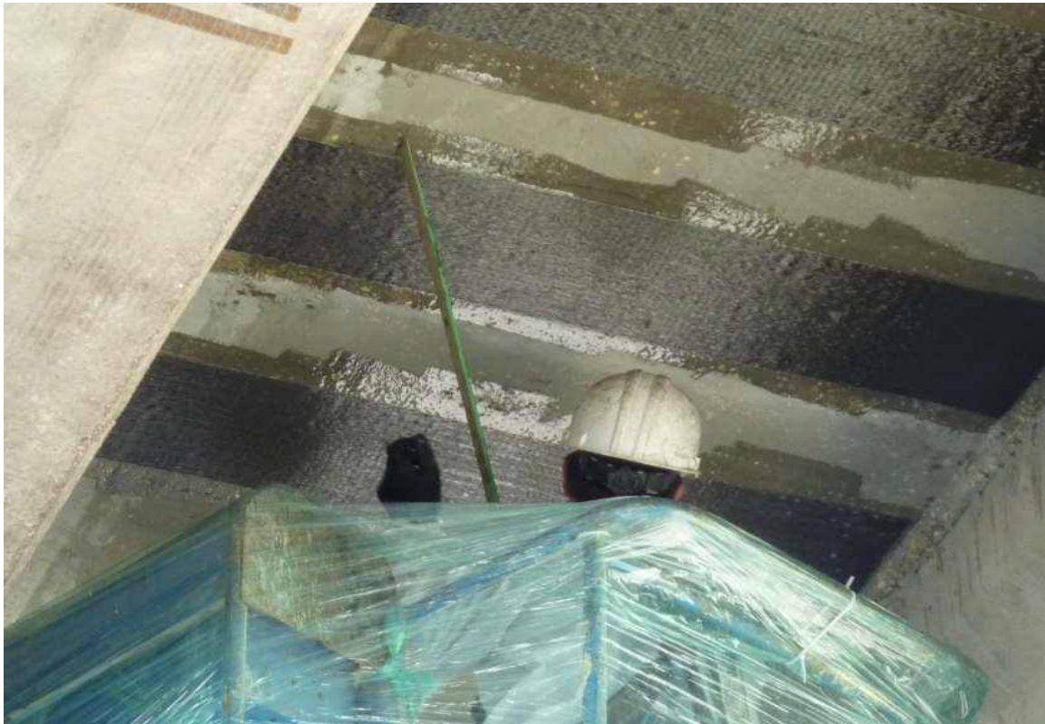
Figure 2.8: Deck Strengthening of Bridge Using CFRP (Shahawy, 2010)
