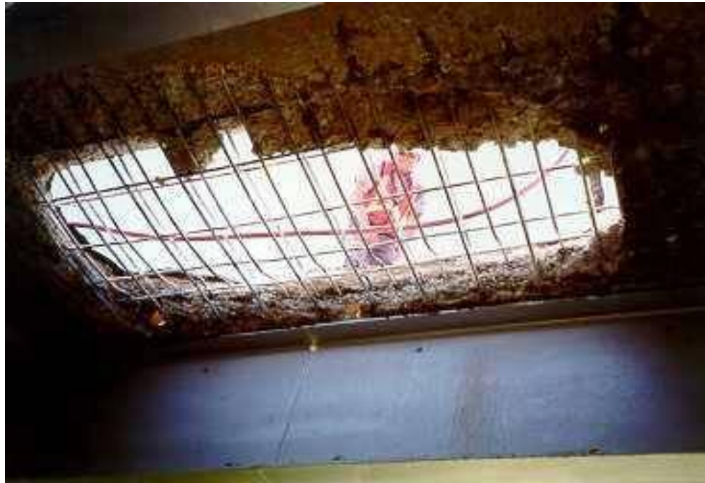
Figure 1.3: Concrete Deck Deterioration Caused by Environmental Factors (Shahawy, 2010)
