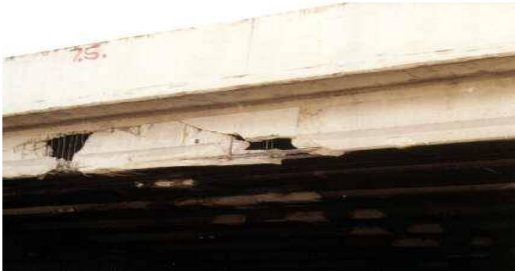
Figure 1.2: Accidental Damage on a Bridge (Shahawy, 2010)
