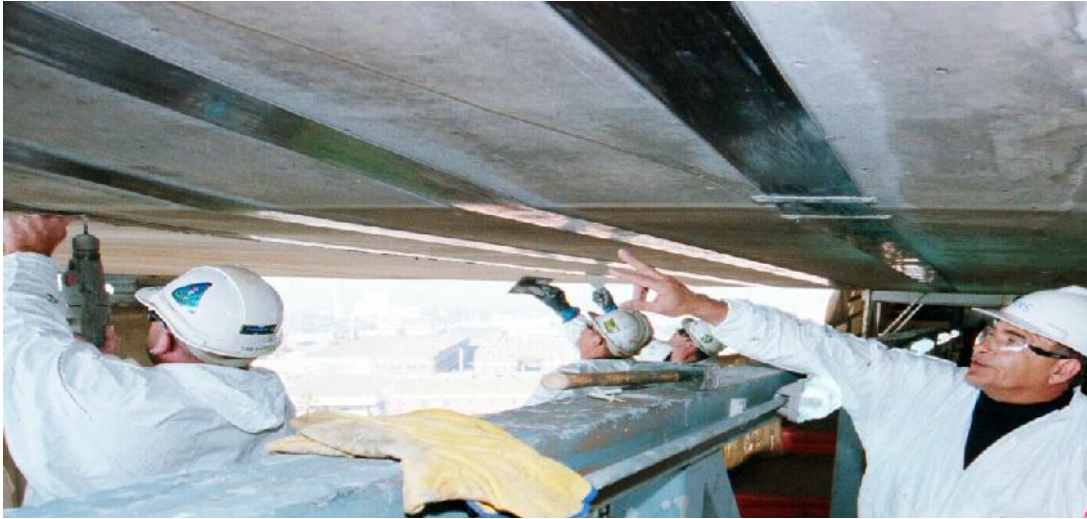
Figure 2.9: CFRP Laminates Strengthening of a Box Girder (West Gate Bridge) (Irwin and Rahman 2002)
