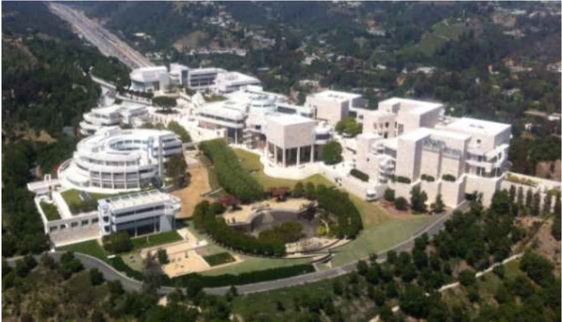
Resim 4.5: Getty Center Binası ( http://www.elitehelicoptertours.com/wp-content/uploads/2012/05/photo-23.jpg )
