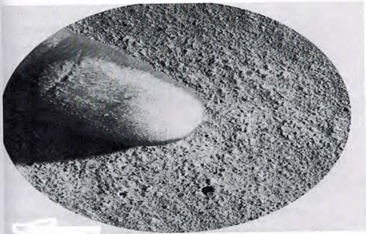
Figure 2.1: Floor Slab Dusting Caused by Carbonation of Fresh Concrete
