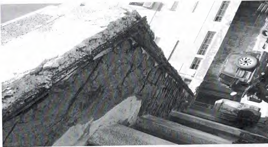
Figure 2.5 c: Reinforced Concrete Corrosion Expected Due to Carbonation
