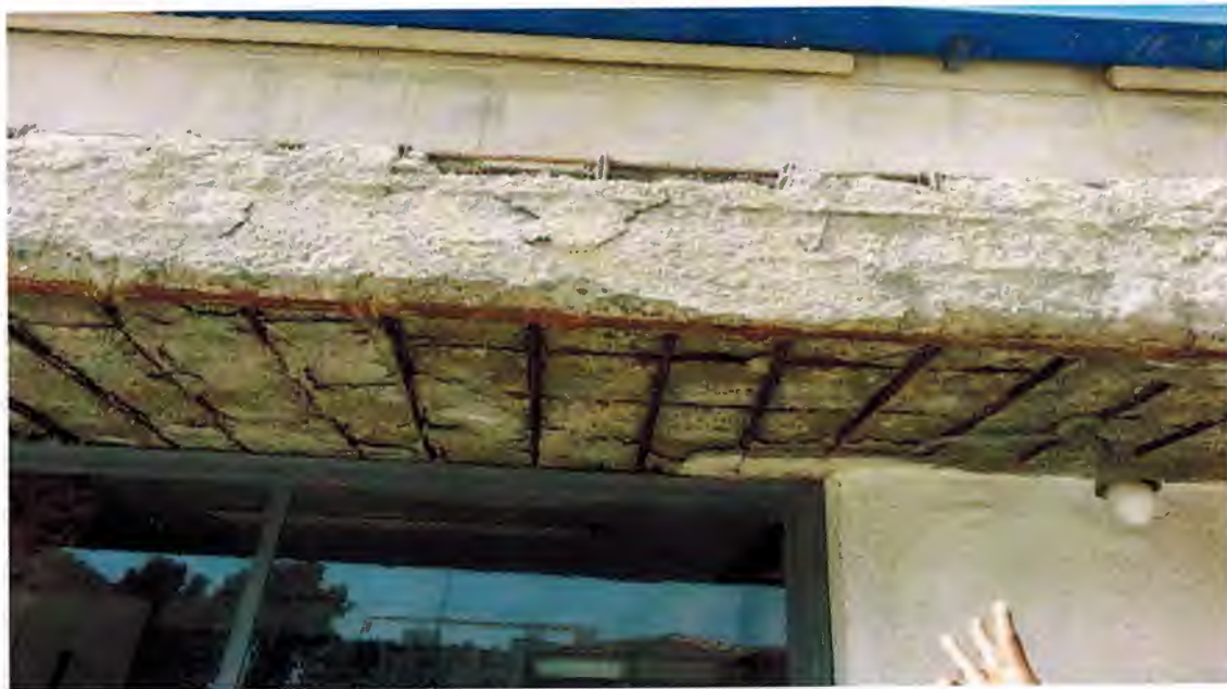
Figure 2.5 b: Reinforced Concrete Corrosion Expected Due to Carbonation
