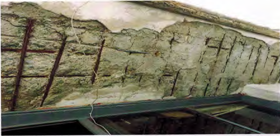
Figure 2.5 a: Reinforced Concrete Corrosion Expected Due to Carbonation
