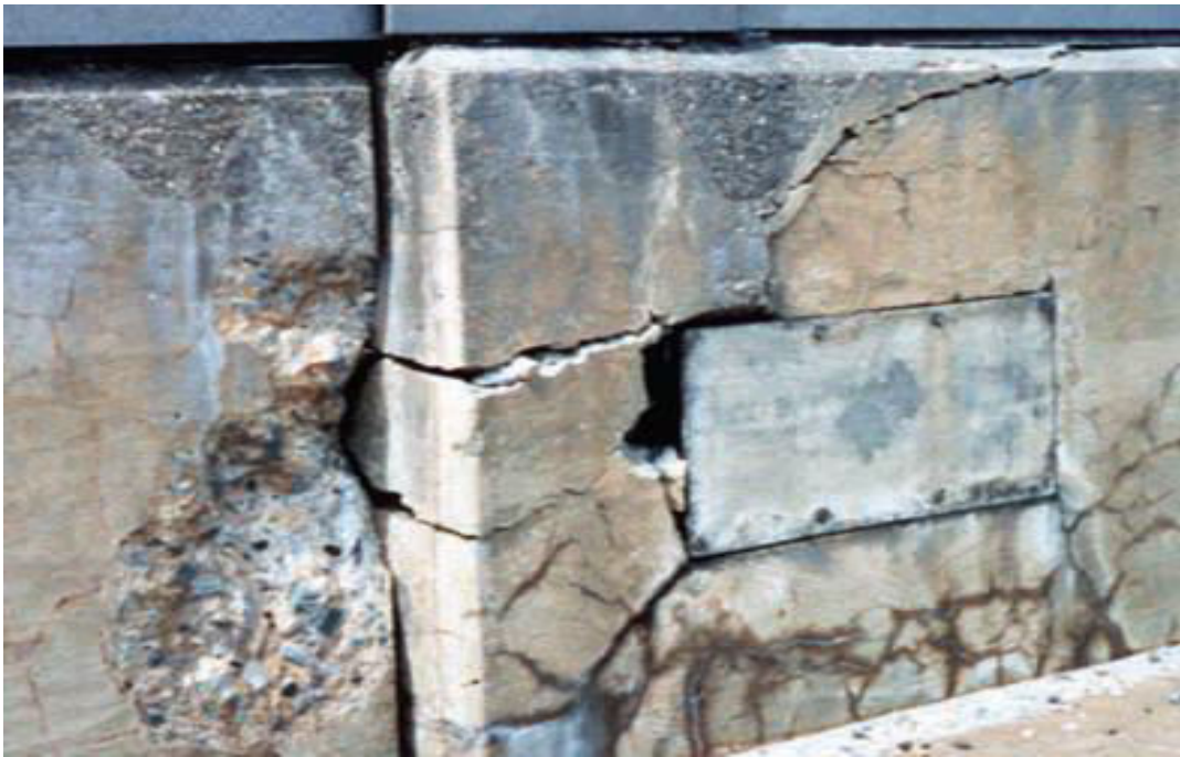
Figure 3.1.2: Parapet Wall affected by ASR (Stark, 1991a).
