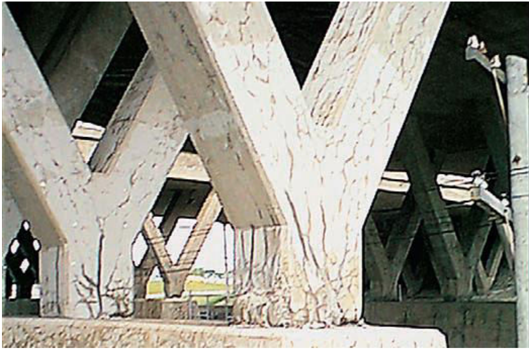
Figure 3.1.3: Cracking associated with stress directions. Predominant cracks are oriented longitudinally in this column (Liu, 1981).
