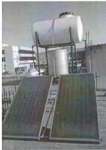
**Figure 2.6:** Typical Application of Tower-Type Solar Water Heater Installed on Flat Roof
