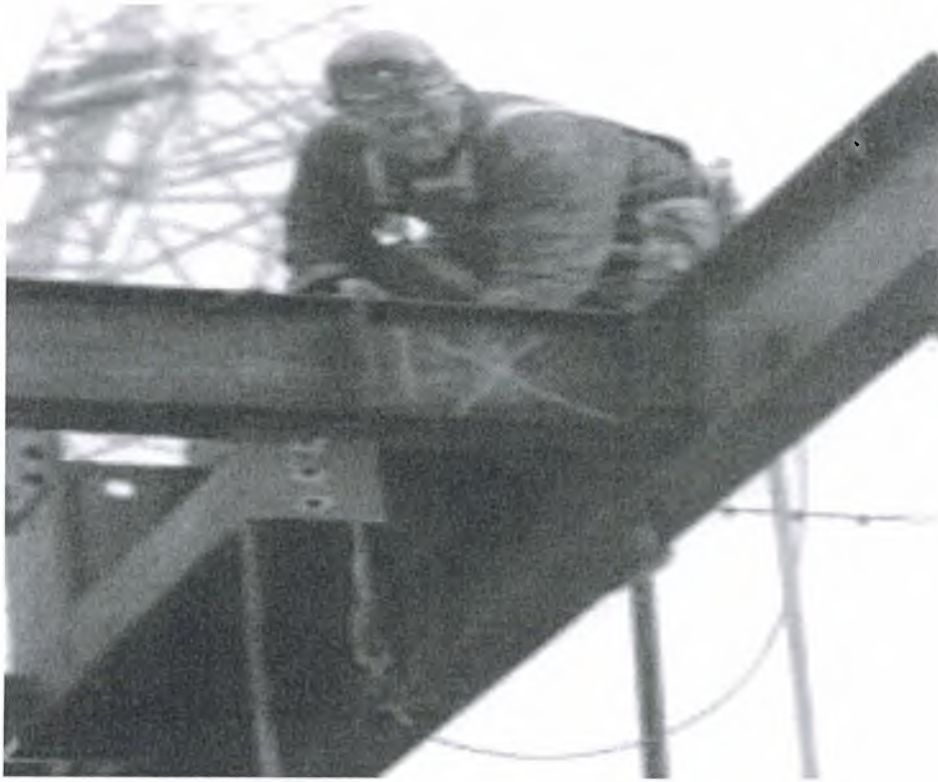
Figure 4.2: Typical Fall protection (Oregon OSHA, 2011)
