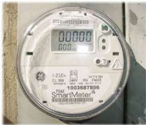
(a) A typical residential smart meter
