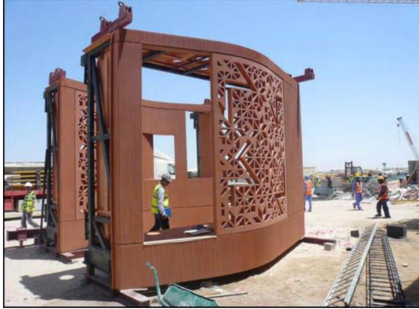
Figure 5.28: Precast façade before fixture to the building (Foster + Partners, 2010)
