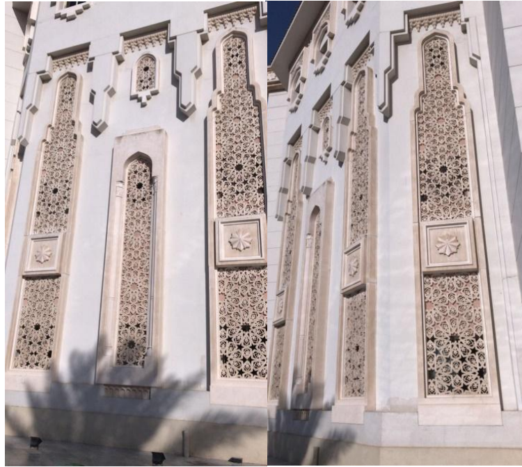
Figure 4.9: Gypsum Mashrabiya used in the Main building at the University of Sharjah (Koujan, 2018)
