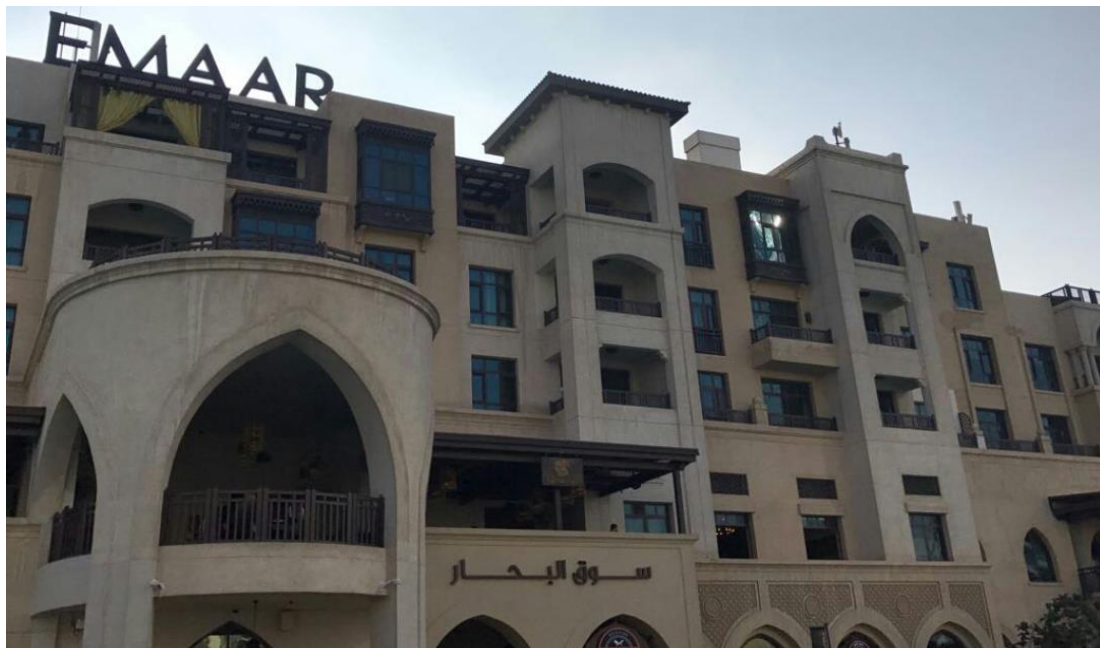
Figure 4.11: Souk Al Bahar in Dubai Mall, using projecting mashrabiya s (Koujan, 2018)
