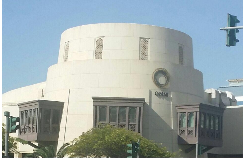
Figure 4.12: Omni Restaurant- Wafi, Dubai using Mashrabiya to cover external openings (Koujan, 2018)
