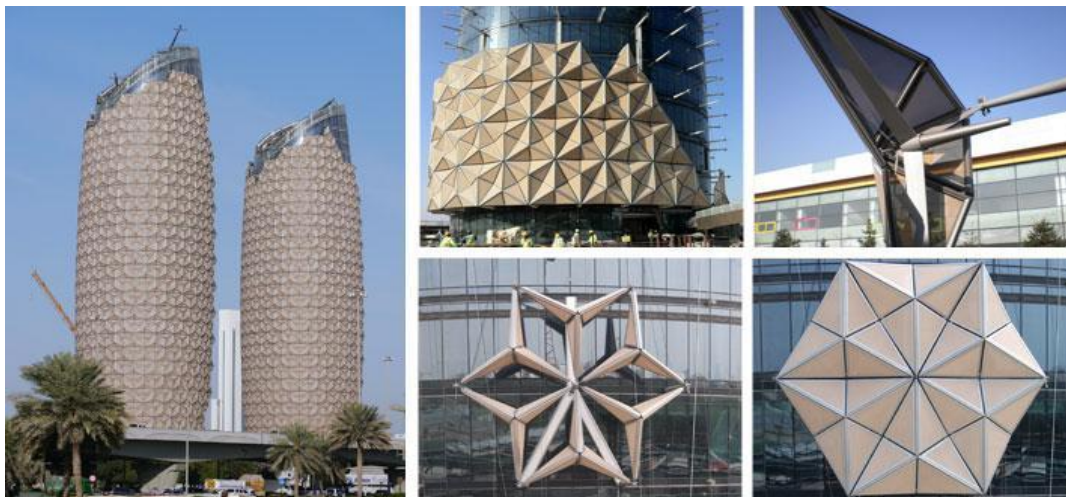
Figure 5.19: Comparison of shading units fully closed left and fully open right
