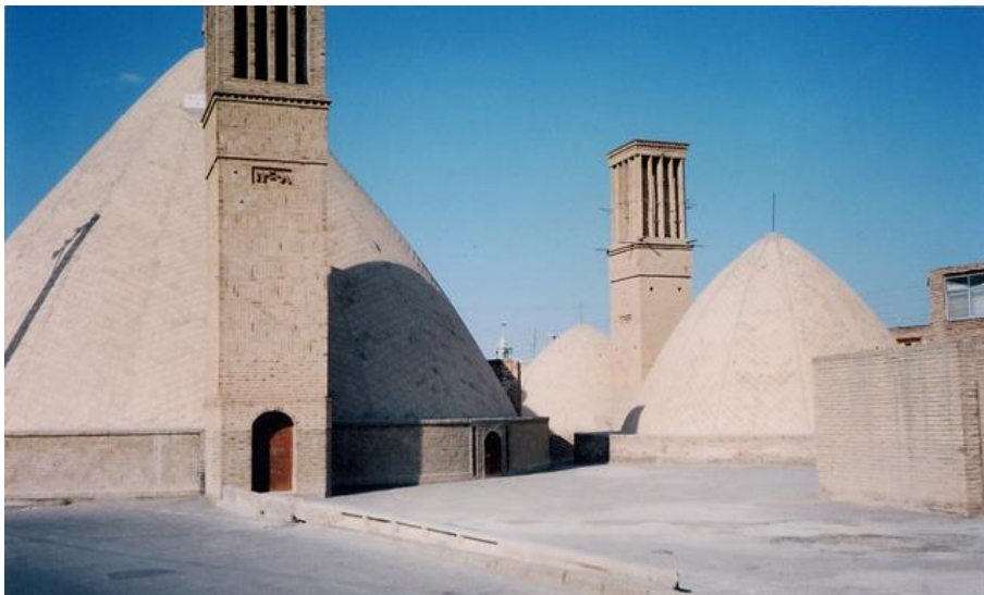
Figure 3.2: Storages with wind catchers in the city of Naeen (Yazd, Iran) (A. A'zami, 2005)
