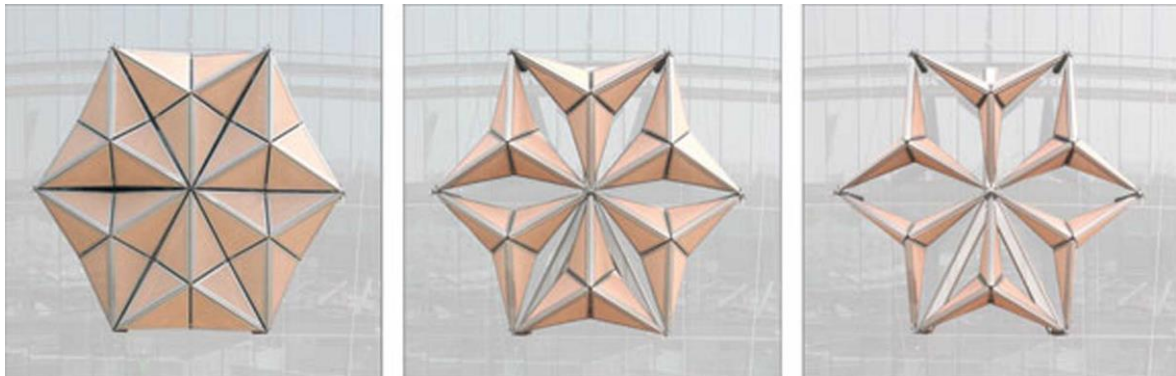
Figure 3.30: Apparent Umbrella-like add-ons that open and close in step with the sun's path (Cook, 2013)
