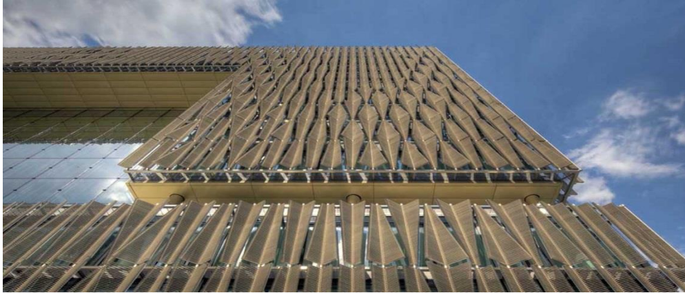
Figure 3.10: Headquarters feather shading system – general view of façade (Arnoldius, 2011)
