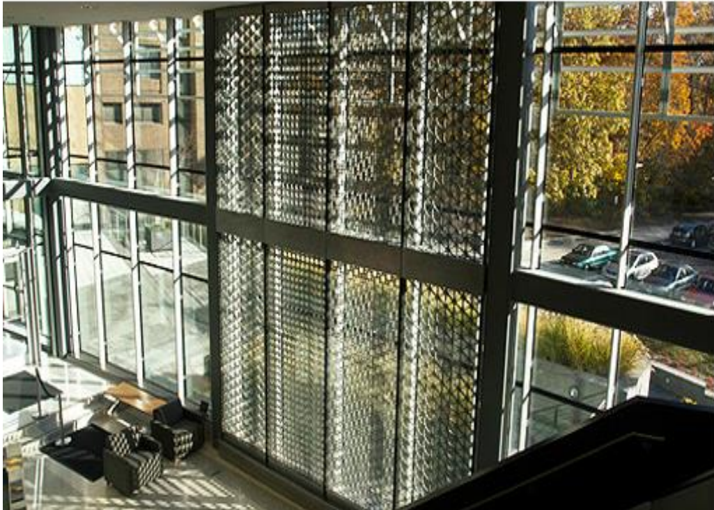
Figure 3.6: Detail of the kinetic surface (Zahner, 2016)
