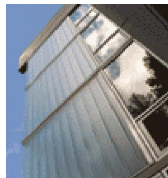
Figure 3.9: U-Channel glass (Buratti, 2013)
