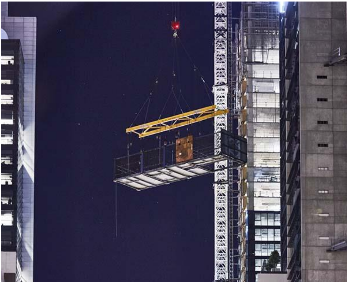
Figure 3.53: Crane hoisting the Hickory's HBS Module in place (Hickory Group, n.d.-a)
