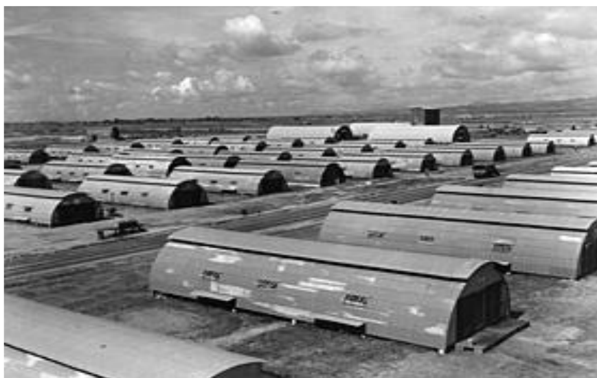
Figure 2.8: Typical Quonset huts built during WW.II (Winding Waters, n.d.)
