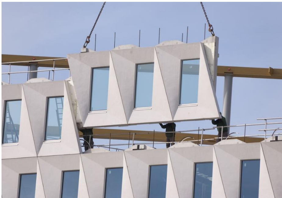
Fig. 3.4: Wall panel of a panelised construction (McGregor, 2017).
