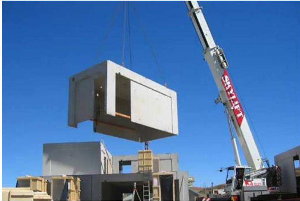
Figure 3.29: Precast concrete volumetric/ modular/3d unit (Green Precast Modular, 2010)
