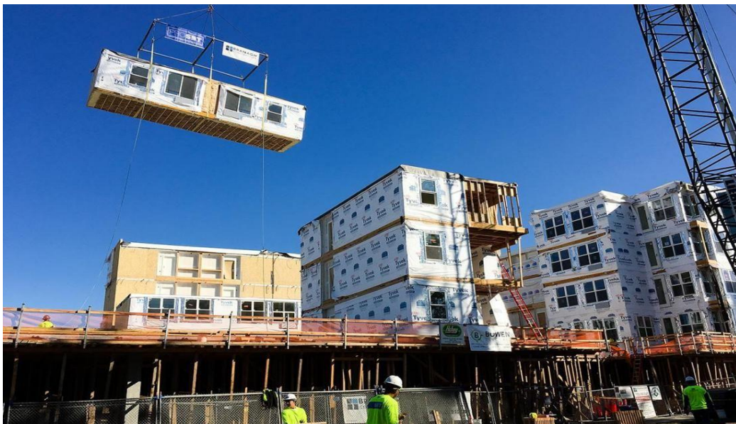
Fig. 3.6: Stacking of a modules at a modular site (Littman, 2017)
