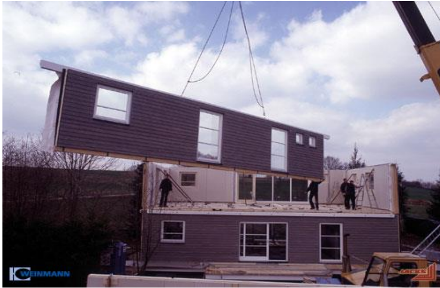
Figure 3.31: Assemblage of a timber panelised wall on site (Jacks New Zealand, n.d.)
