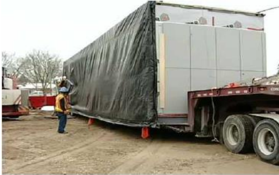
Fig. 3.10: Typical completed volumetric module ready to be transported to site from the factory (Velamati, 2012)
