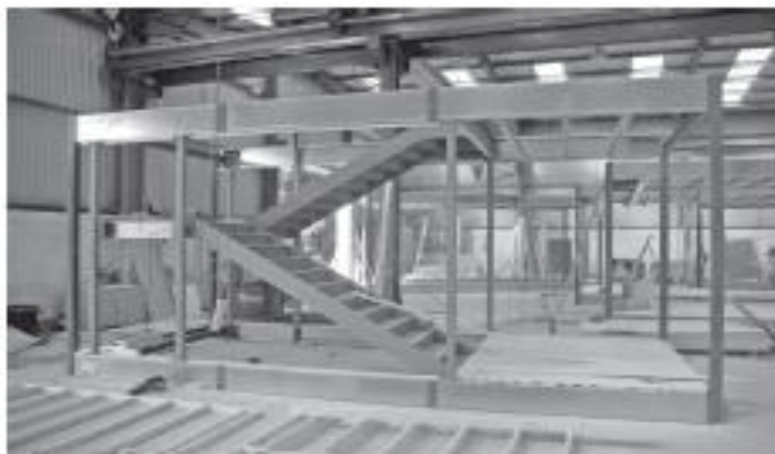
Figure 3.22: Stair module with corner posts (Steel Construction Info, n.d.)
