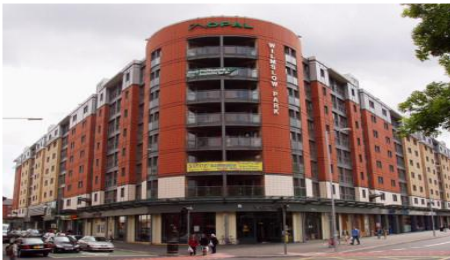
Figure 3.20: Typical modular structure supported by a primary concrete podium (Lawson & Ogden, 2008)
