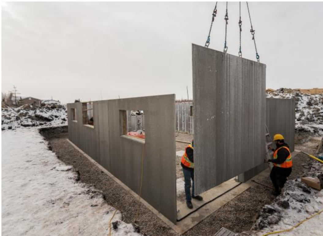
Figure 3.1: Precast concrete walls being craned to position (Superior Walls, 2016)
