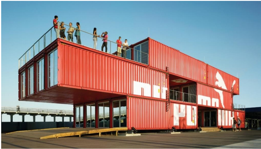
Figure 3.23: Typical building structure made from series of modular shipping containers (Belogolovsky, 2018)
