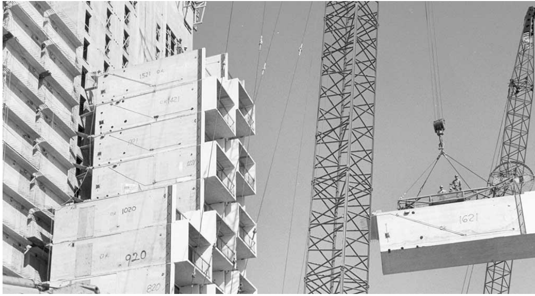
Figure 2.10: A crane hauling a module in place during construction of the Hilton Palacio Del Rio Hotel (1968) (Zachry Construction, n.d.)
