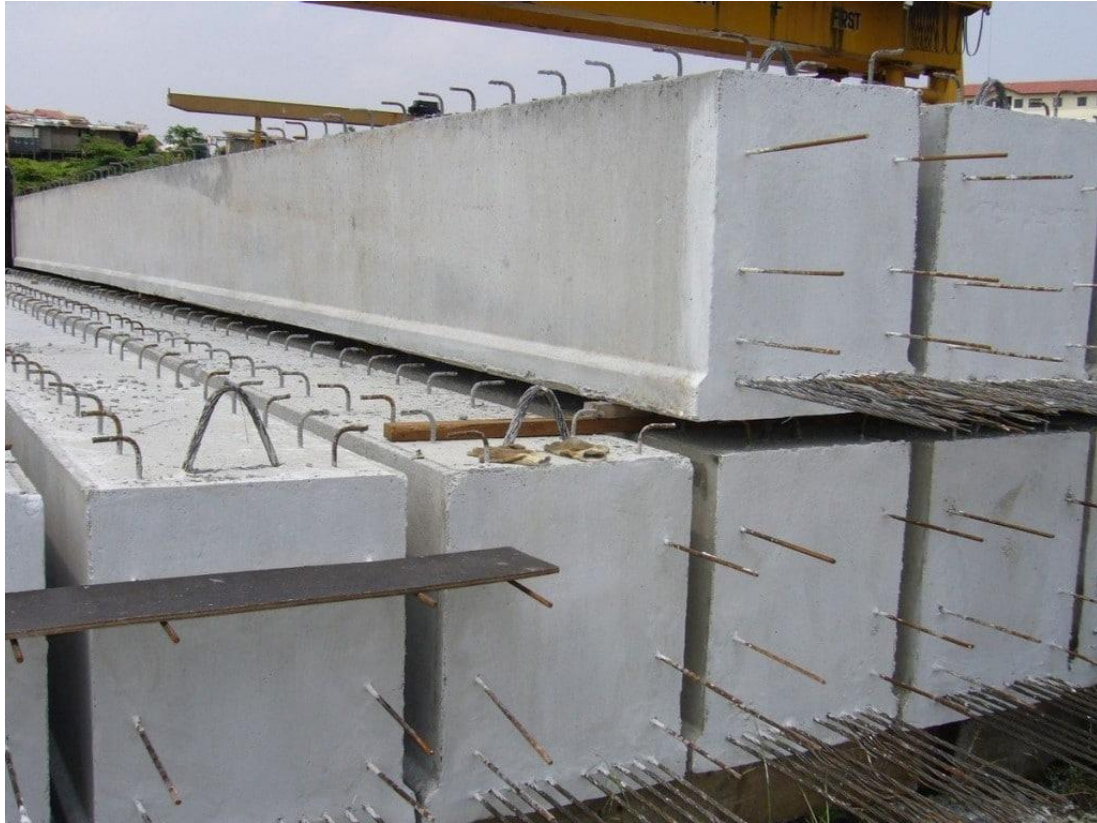
Fig. 3.2: Pre-stressed concrete elements (The Constructor, n.d.)
