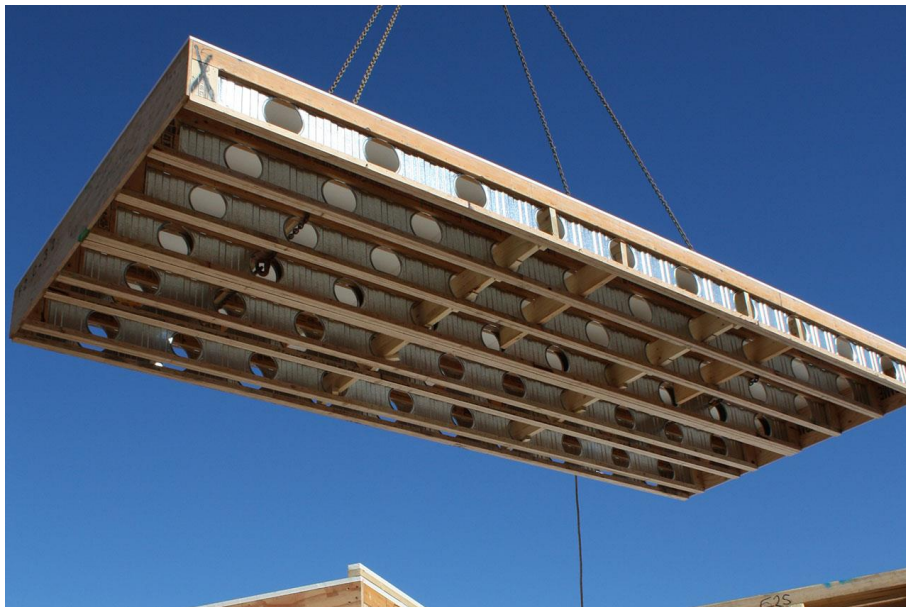
Figure 3.32: Timber floor/ceiling panel (Colli Timber & Hardware, n.d.)
