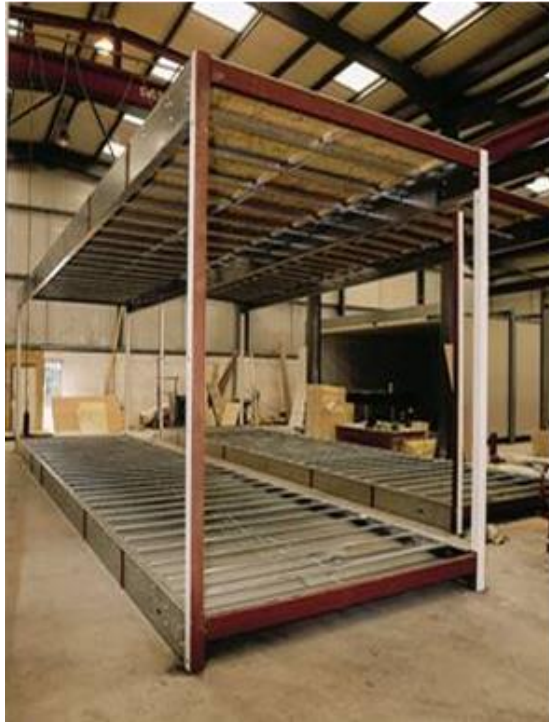
Figure 3.14: Primary steel frame used in open-sided module (Steel Construction Info, n.d.)
