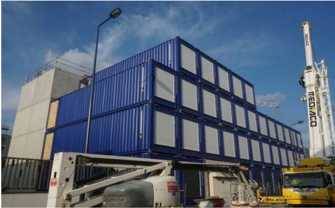
Figure 3.60: Module of the Container Student Housing being stacked (XCUBE Engr & Prefab, 2015)
