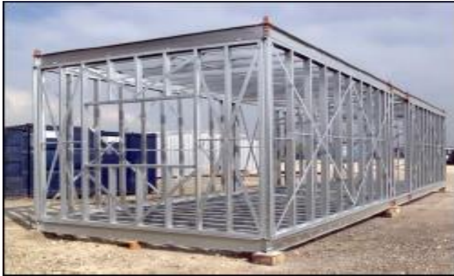
Figure 3.15: Partially open-sided module, (Lawson & Ogden, 2008)
