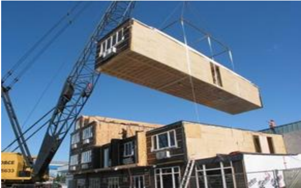
Figure 3.5: Stacking of a modules of a modular structure (WM Modular, 2017)
