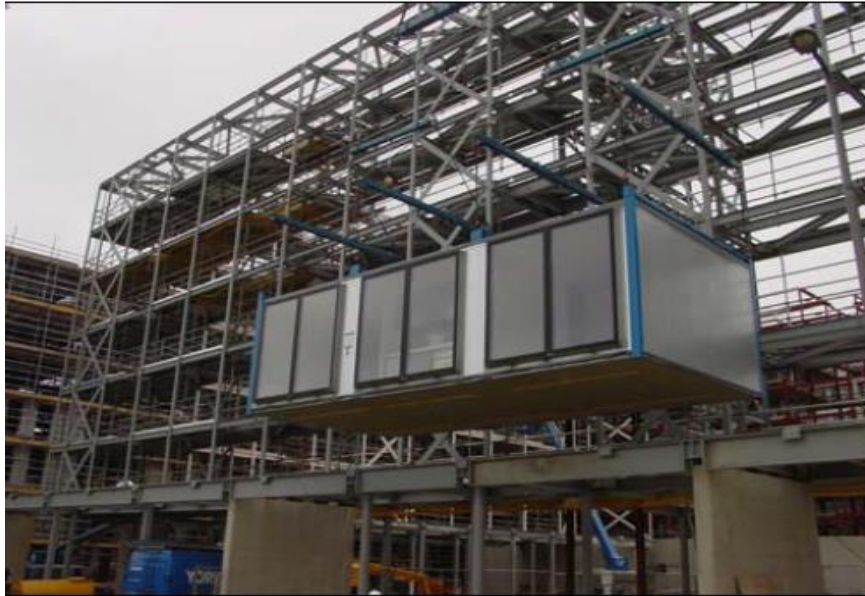
Figure 3.19: Installation of modules supported by a primary steel structural framework at MoHo, Manchester (Steel Construction Info, n.d.)
