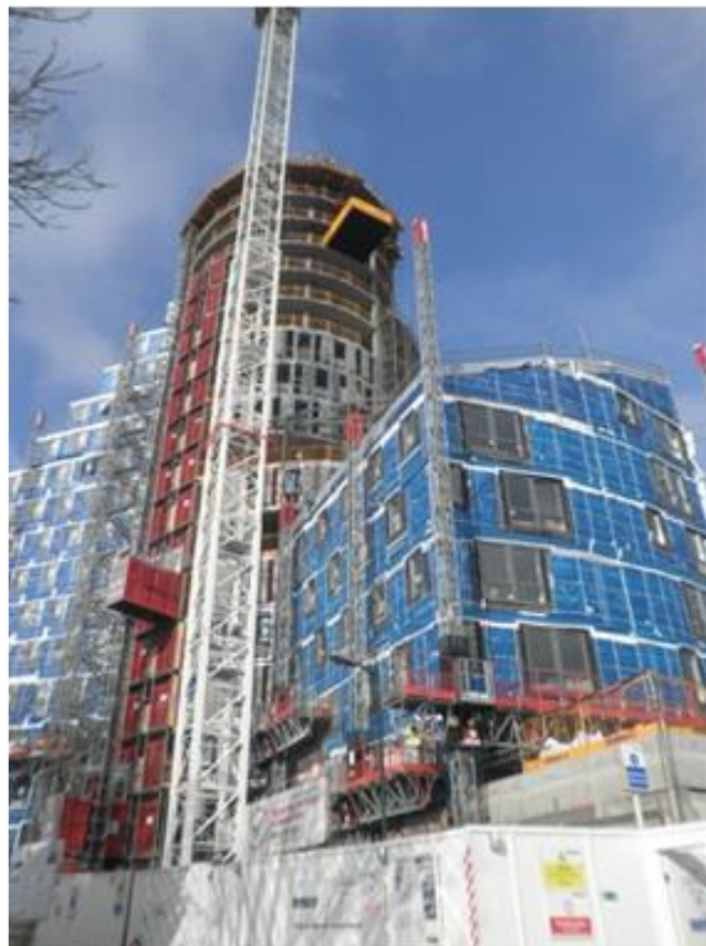
Figure 3.26: Hybrid modular system using skeletal structure (MBI, 2013)
