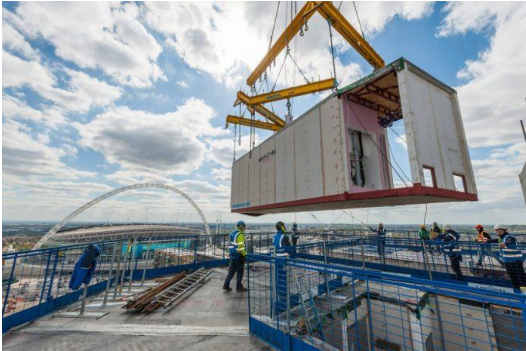
Figure 3.42: Modules for the Apex house being hoisted into position with a crane (Digital Construction News, 2017)
