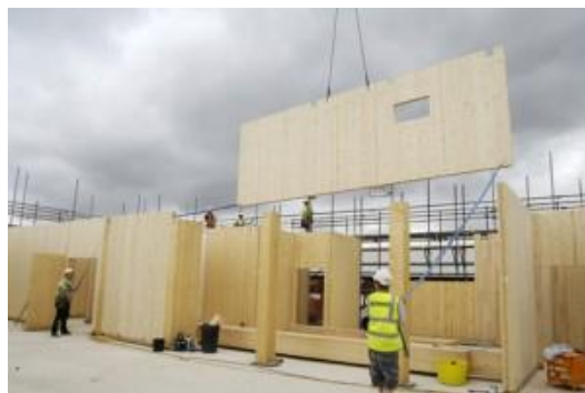
Figure 4: CLT – Cross laminated timber being installed (SCS, 2013)
