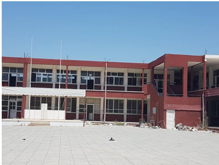
Figure 3.1: Bayraktar school before demolition, Nicosia, North Cyprus.
