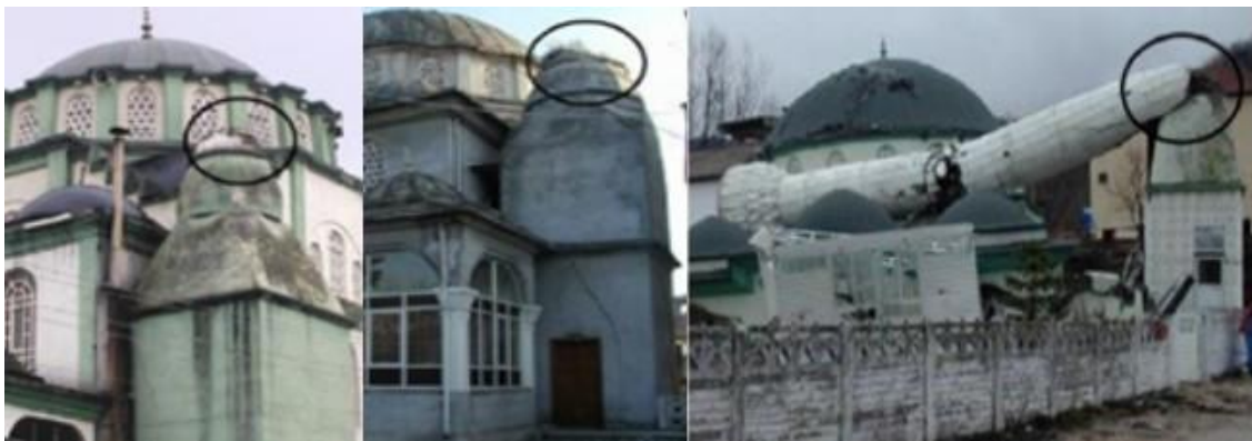
Figure 1.7: Minarets collapsed during Kocaeli and Düzce earthquakes (Sezen et al., 2008)
