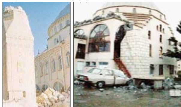
Figure 1.4: The collapsed minarets in Erdemli, Mersin, Turkey (Türkeli, 2014)
