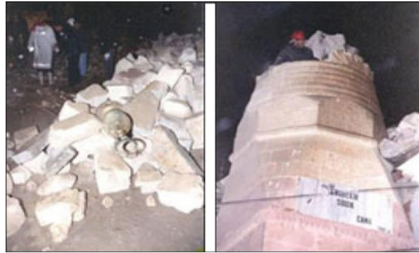
Figure 1.3: The collapsed minaret of the Ebubekir Sıddık Mosque, Kayaş, Ankara, Turkey (Türkeli, 2014)
