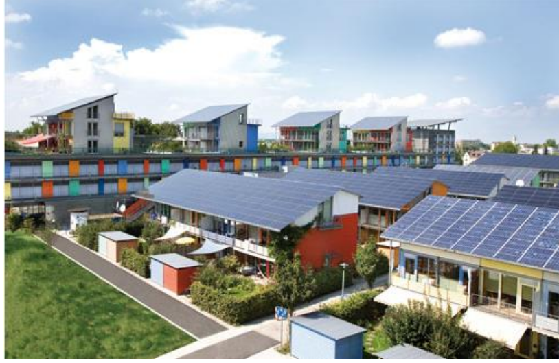
Şekil 4.20: Binalardaki Güneş Panelleri, Freiburg ( http://www.ecotippingpoints.org/our-stories/indepth/germany-freiburg-sustainability-transportation-energy-green-economy.html )
