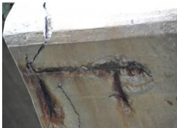
Figure 2.5: The impact of reinforcement corrosion on concrete (Zonneveld, 2015)
