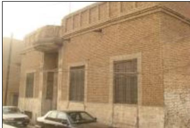
Figure 3.17: The facade of the building demonstrated exposed burnt brick (Kareim, 2018)
