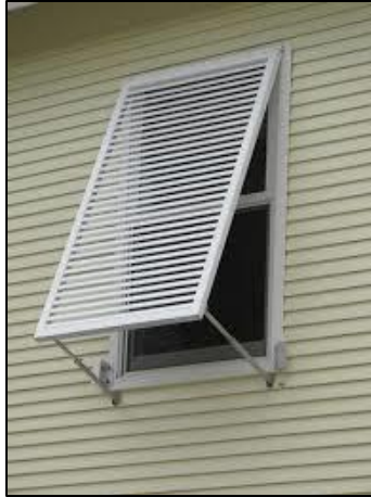
Figure 2.5: Shade screen for absorbing direct solar radiation (Lstiburek, 2004)
