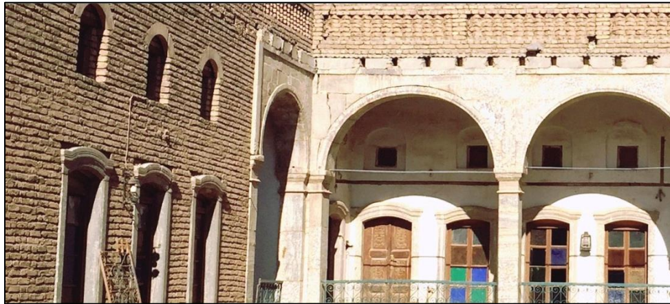
Figure 3.13: Windows facing courtyard for stack and cross- ventilation (Kareim, 2018)
