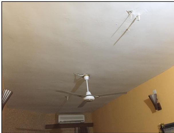
Figure 3.25: The slab from inside covered by gypsum plastering (Kareim, 2018)
