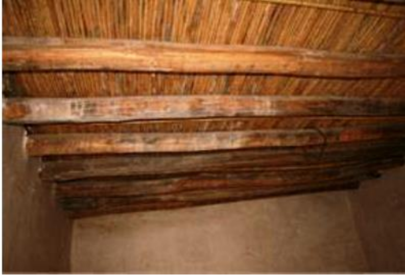
Figure 3.9: Roofs boarded with wooden planks (Kareim, 2018)
