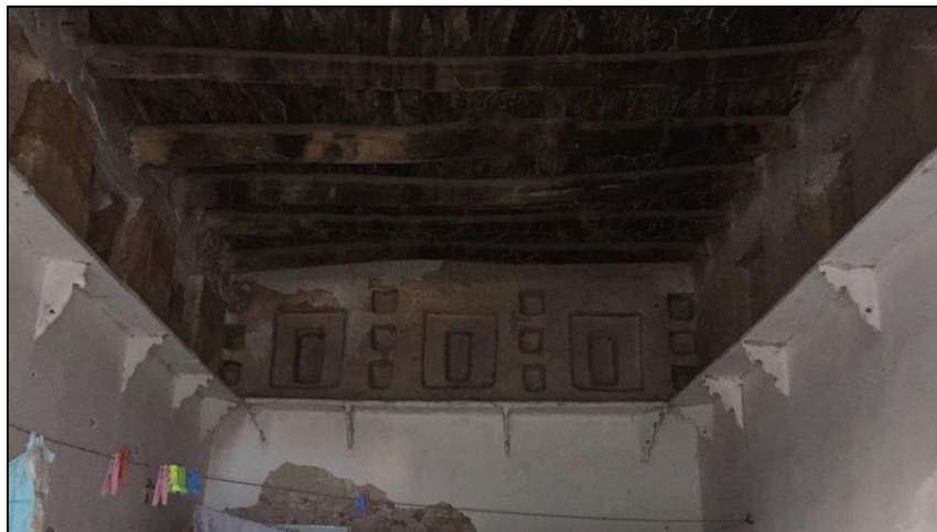
Figure 3.22: Roof of the building made by wood, burnt brick and clay (Kareim, 2018)
