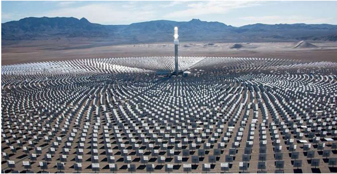
Figure 2.10: Central receiver(Environmental and Energy Study Institute (EESI), 2009)
