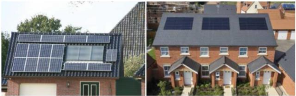
Figure 3.18: Add solar modules to sloping surfaces above external finish materials (Sinapis & Donker , 2013)
