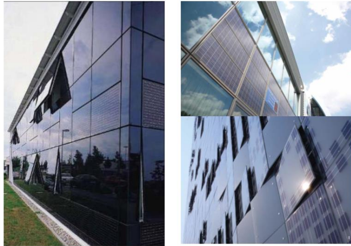
Figure 3.22: Solar Cells on Building Facades (Krawietz, 2011)
