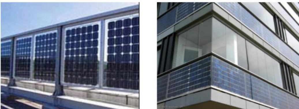
Figure 3.26: Solar cells for handrails (Krawietz, 2011)
