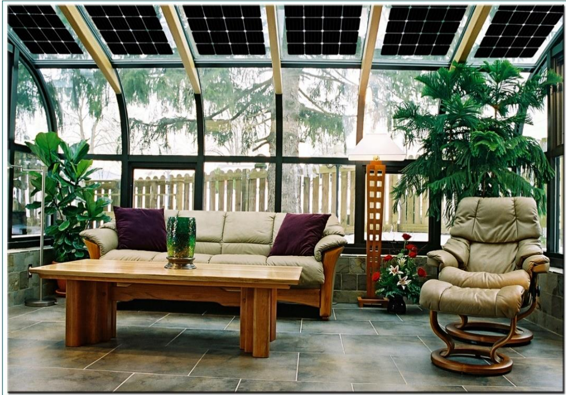
Figure 3.16: Solar modules used as natural roof lighting
