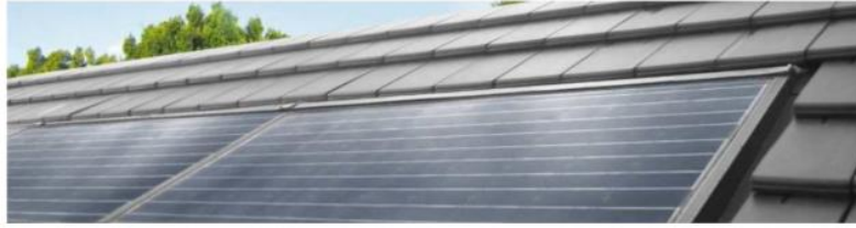
Figure 3.17: Solar modules are used in place of the original surface finish materials (Sinapis & Donker , 2013)
