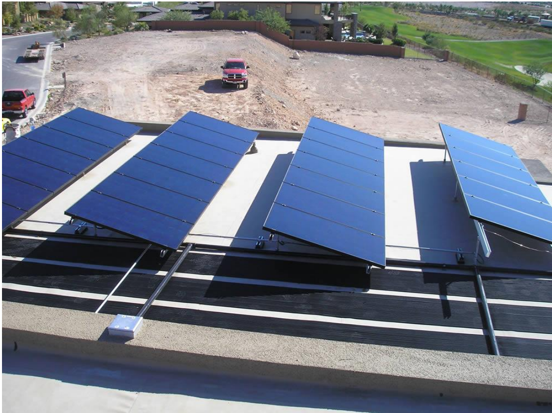
Figure 3.14: Sloping solar modules designed for horizontal surfaces (bombard, 2015)
