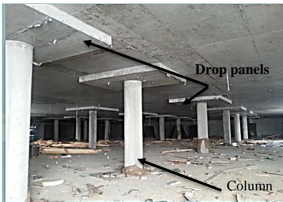
(c) Flat slab with drop panel
