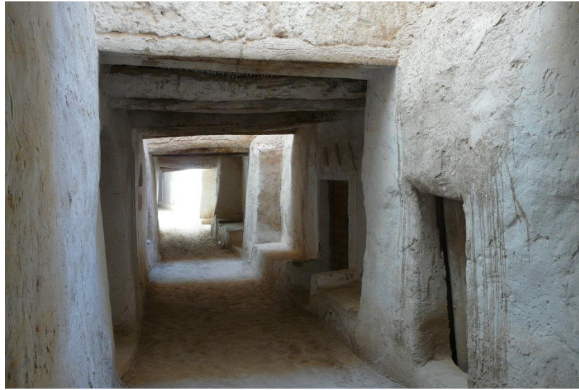
Figure 4.2: Traditional Ghadames houses showing connected walls, passage ways, and entrances
