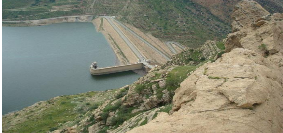
Figure 3.3: Darbanikhan construction project (Author, 2019)
