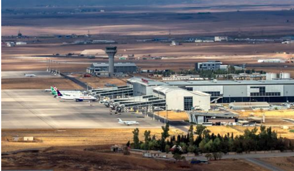
Figure 3.1: Mosul Airport construction project (Author, 2019)
