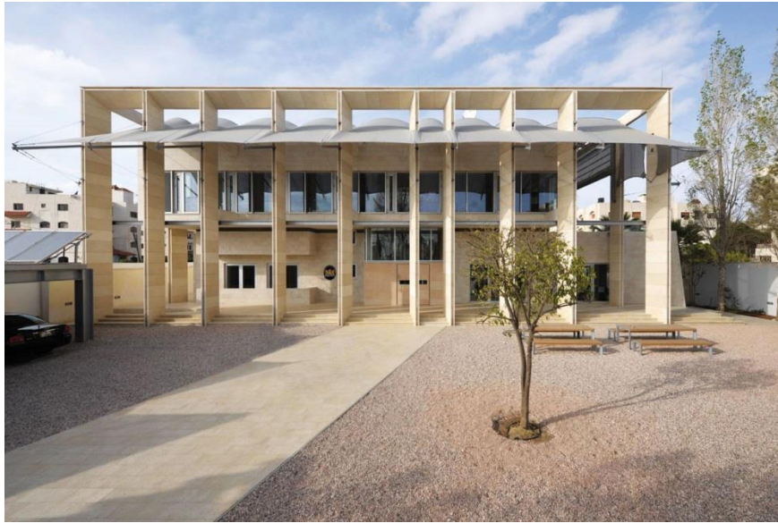
Figure 4.8: Front elevation with colonnade and shading of the Dutch Embassy Building in Amman (Al-Azhari & Al-Najjar, 2012)
