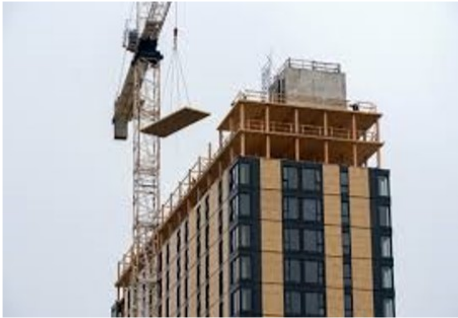
Figure 4.6: The Brock Commons Residence under construction ( www.canadianarchitects.com , 17February 2019)
