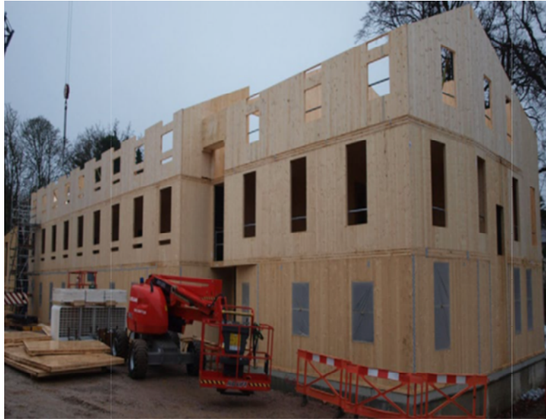
Figure 3.14: Platform construction (Chulain, 2016)
