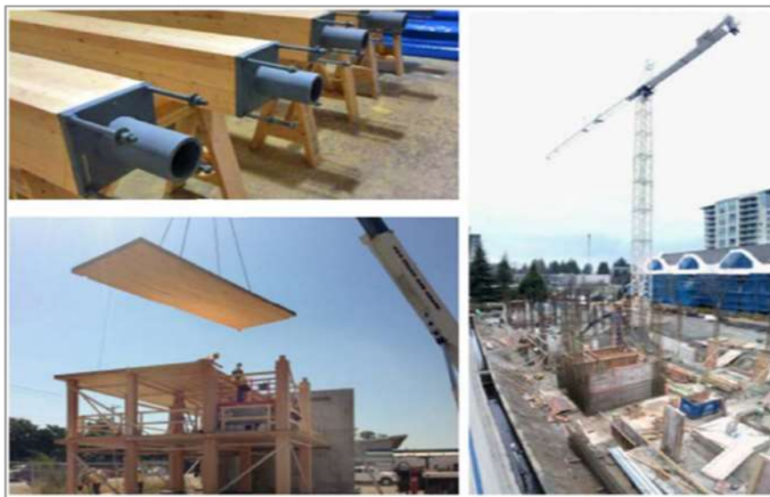
Figure 3.9: CLT mass timber used in construction site (Style Architects, 2016)
