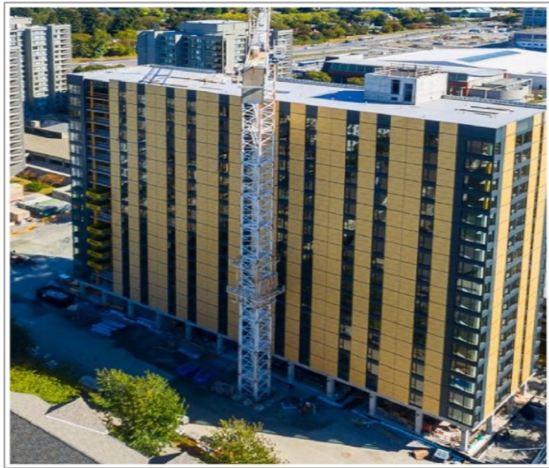
Figure 4.5: The UBC CLT mass timber construction ( www.archdaily.com/office/acton-ostry-architects )
