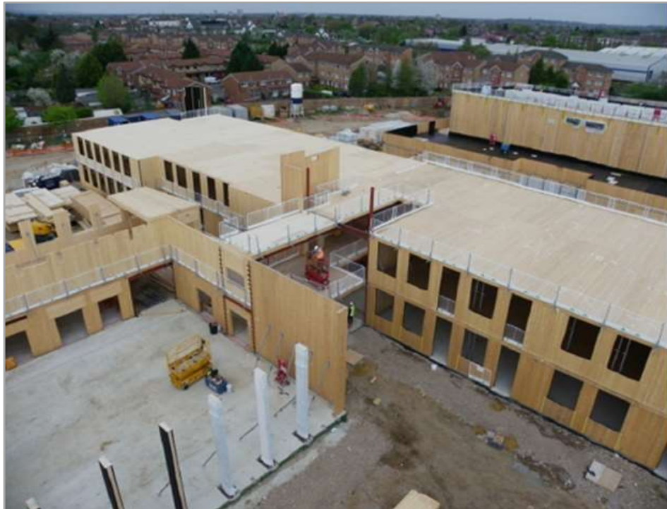
Figure 4.3: The construction of Mayfield school, UK (Hartmann, 2015)
