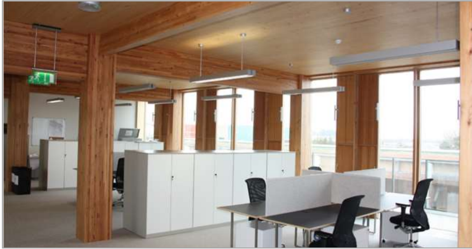
Figure 3.16: CLT mass timber used as a roofing system ( www.holmesstructures.com )
