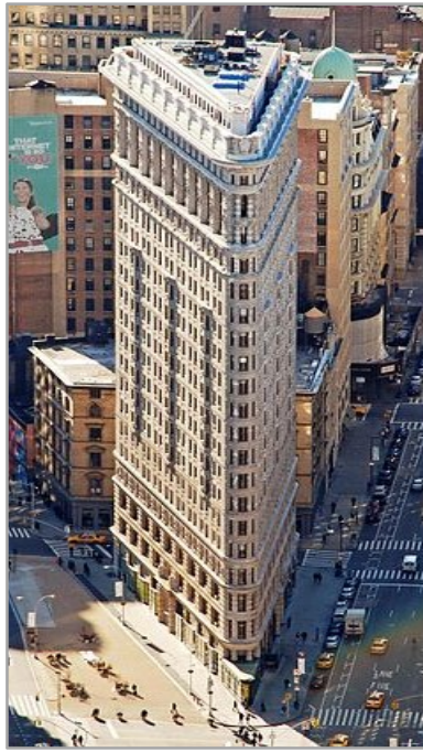
Figure 2.6: Flatiron Building built in 1902 ( www.skyscrapercenter.com )
