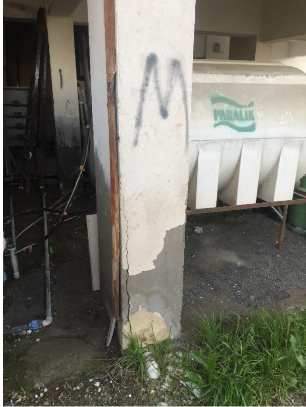
Figure 5.4: Observed cracks on column
