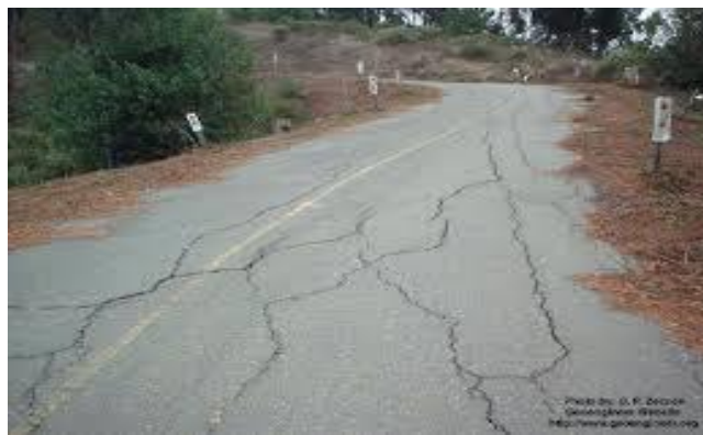
Figure 1.3: Expansive soil in road Colorado, USA (Nelson, 1997)
