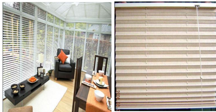
Figure 2. 15: Internal shading devices (Improving the Thermal Performance of the Building Envelope, 2016)
