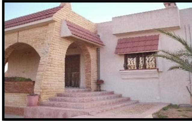
Figure 4.38: The windows made from PVC and steel
