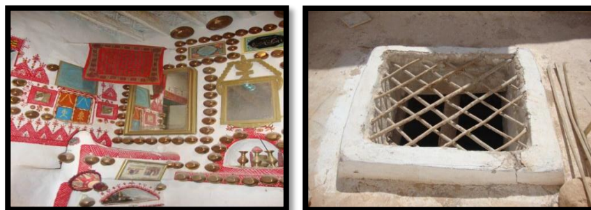
Figure 3.8: The mirrors reflecting natural light into the rooms, and windows is opening at the roof (Shahran, 2018)
