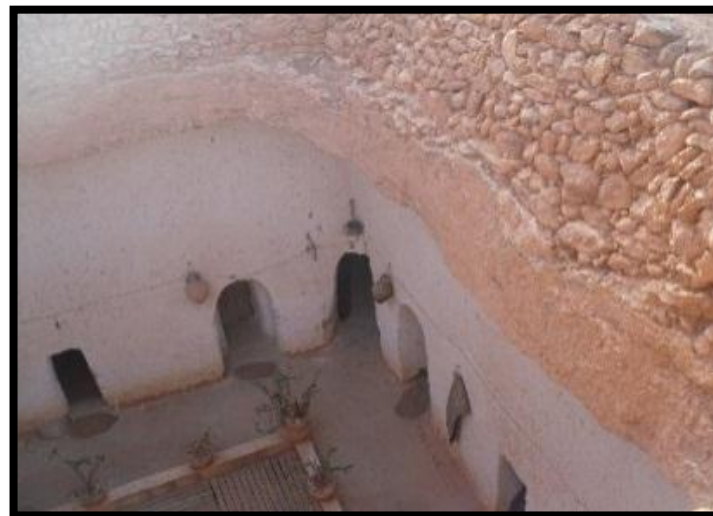
Figure 4.25: The rubble stones were used to prevent soil collapse (photo by author)
