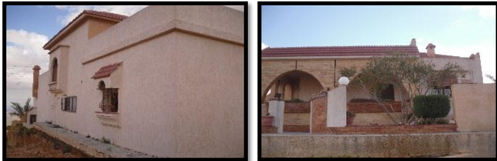
Figure 4.39: The house was painted with normal paint and pharaonic bricks of used in the verandas (photo by author)
