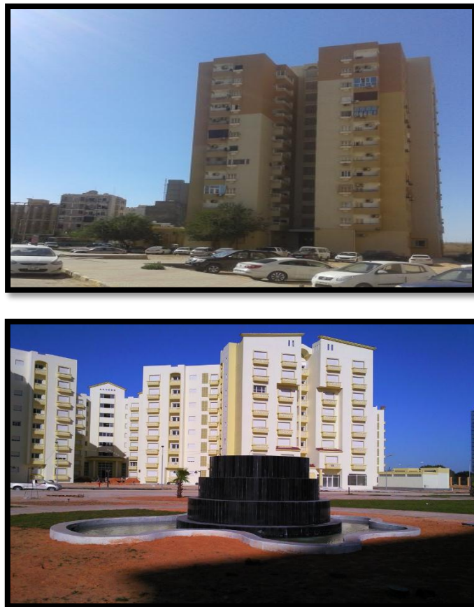
Figure 3.15: The apartment buildings in Tripoli city .Multistory houses ( https://mapio.ne . Last accessed April 2019)
