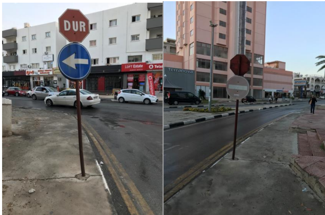
Figure 4.9: Insufficient traffic signs in Ismet Inonu Boulevard
