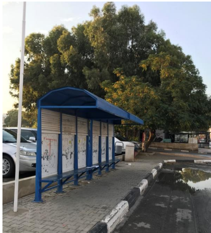
Figure 4.12: Bus station with shelter and bench in Ismet Inonu Boulevard
