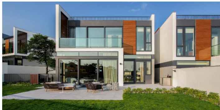
Figure 17: Rear elevation of whitesands housing (SAR, 2011)
