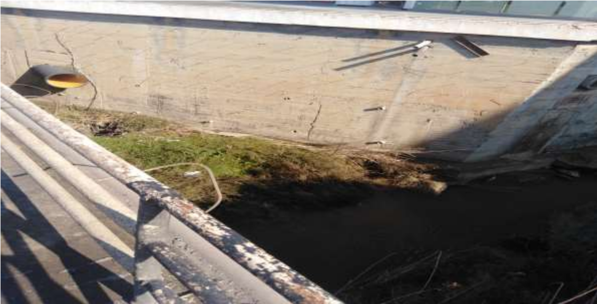
Figure 5. 17: Concert wall, and a runoff discharge is exposed to the river directly, Main Tributary, Kucukkaymakli area –Lefkosa –Nicosia
