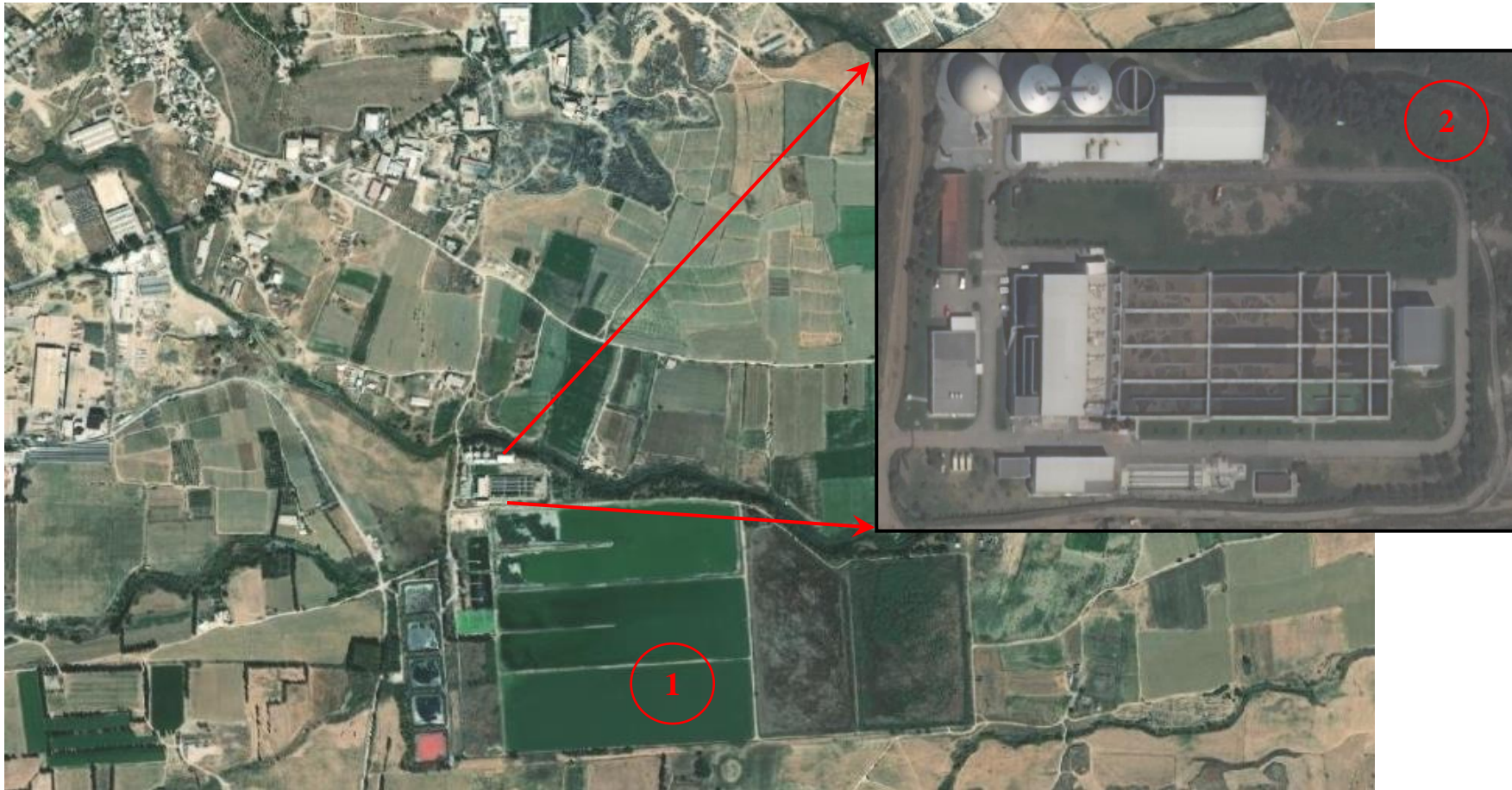
Figure 3. 13: Treatment Plants within NTM boundaries. Number1, old wastewater treatment plant . Number 2 , New wastewater treatment plant (Google, n.d).
