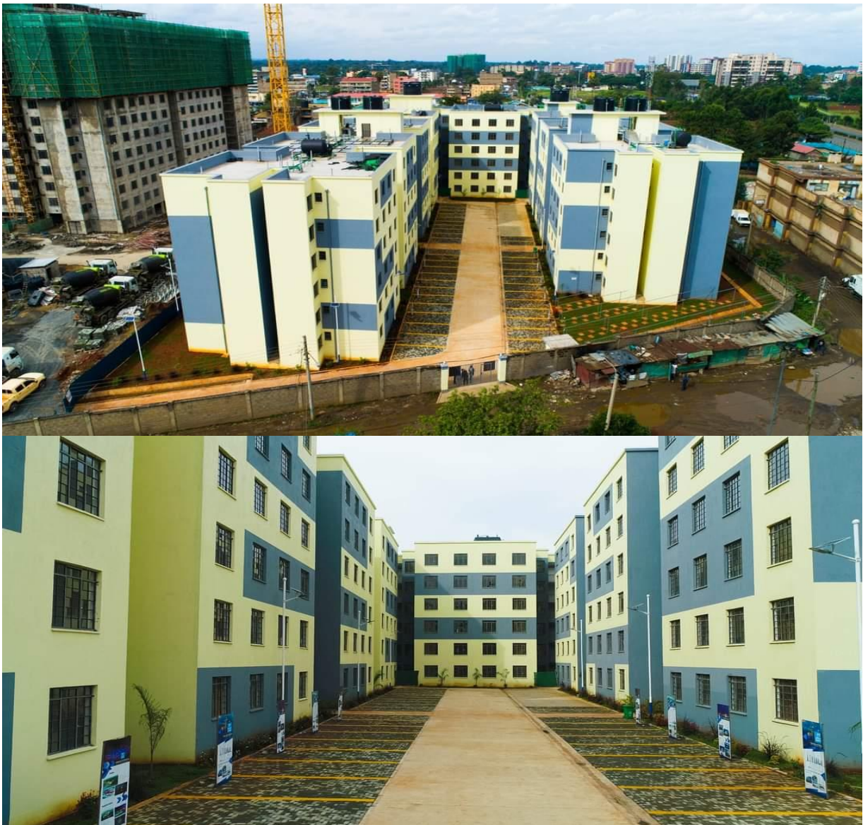
Figure 4.10: Completed Units of the park-road housing program. (Pwk, 2020)
