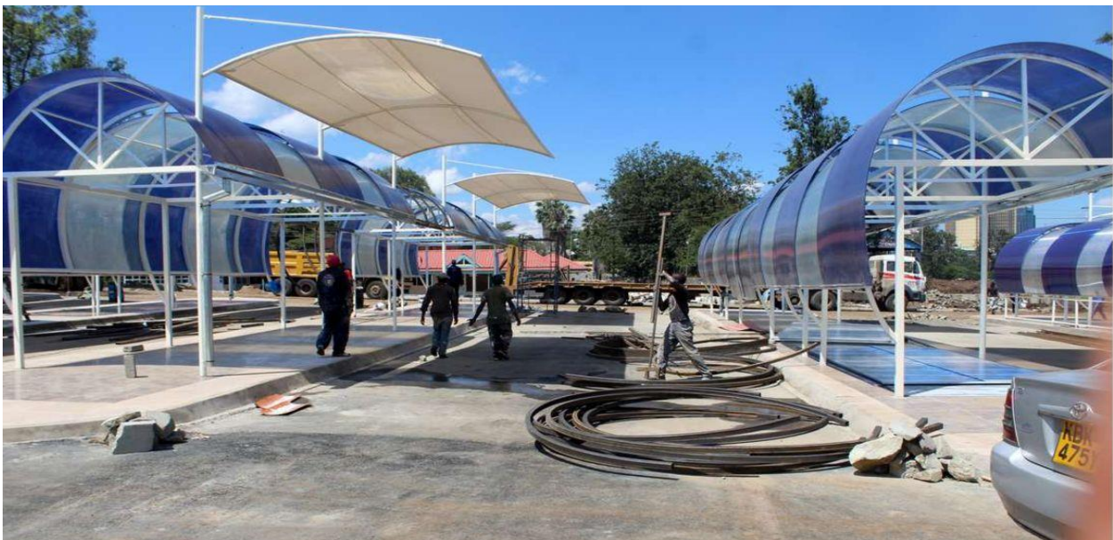
Figure 4.11: Green-park bus terminus ongoing construction. (Nmskenya, 2020)
