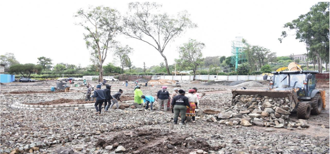
Figure 4.13: Regeneration works on the green-park bus terminus brownfield land (Nmskenya, 2020)
