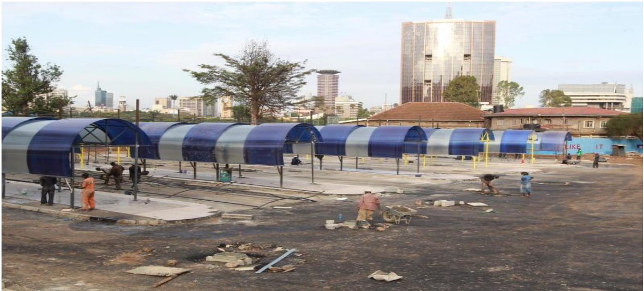
Figure 4.14: Regeneration works on the green-park bus terminus brownfield land (Nmskenya, 2020)
