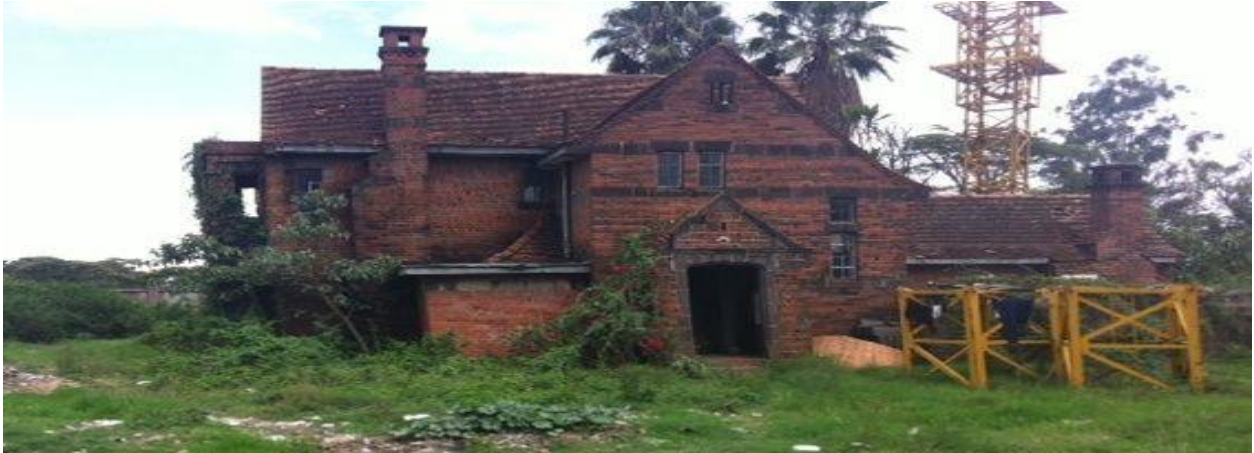
Figure 4.5: Old derelict building in Nairobi.
